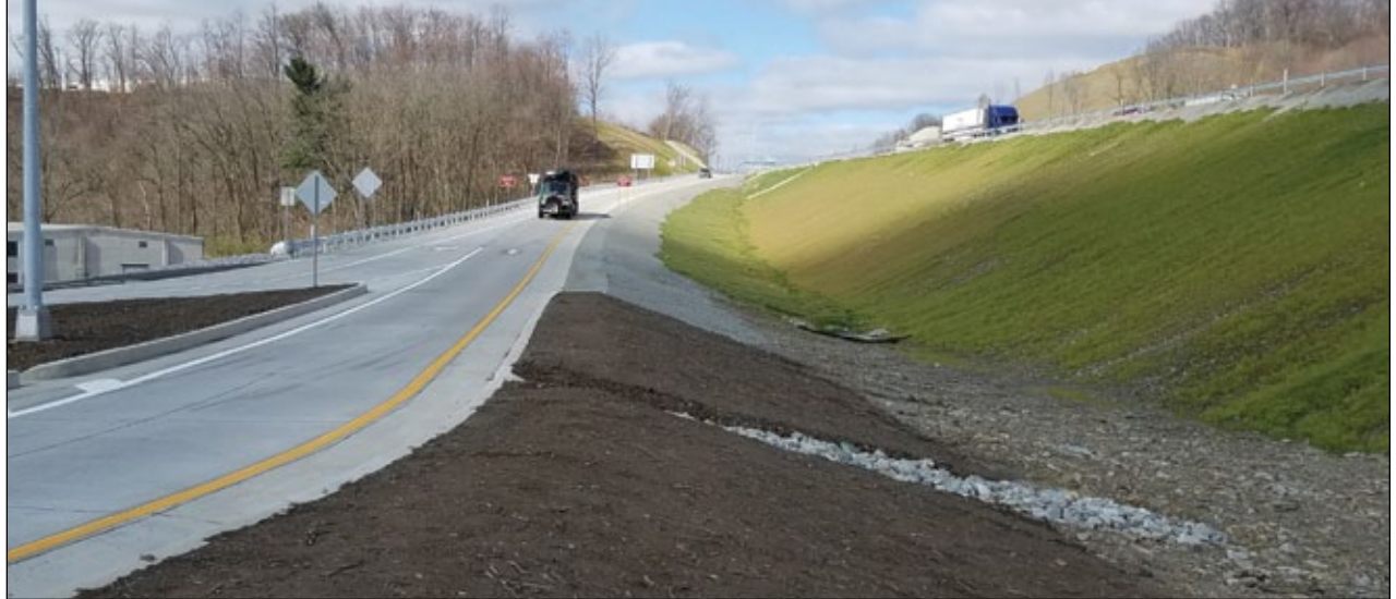
A view of the improved Interstate 70.
