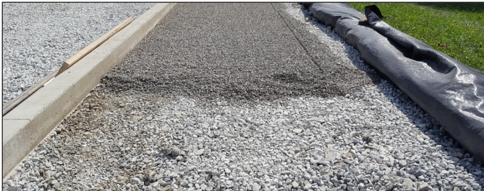
Fabric layer with clean stone placed on top
