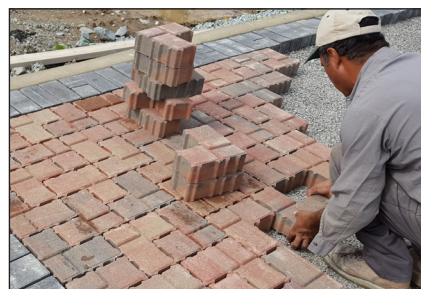
Installing precast concrete pavers.
