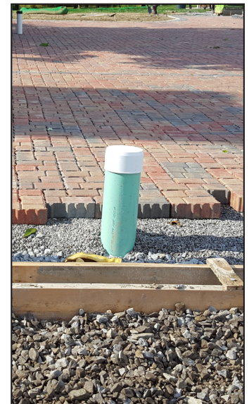
Vertical inspection pipe to be cut off and capped at the surface when paving is completed.
