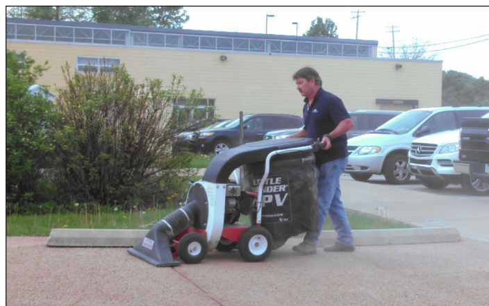
Walking behind the vacuum for permeable paving.
