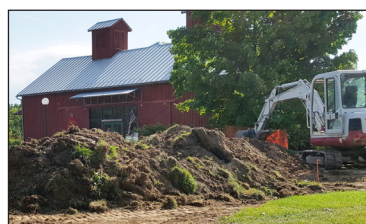
Remove grass and topsoil to create pavement base.
