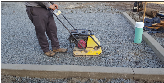
Using a tamper to compact stone layer.
