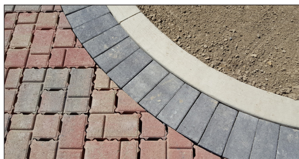
Concrete pavers cut on a curve with a concrete edge
