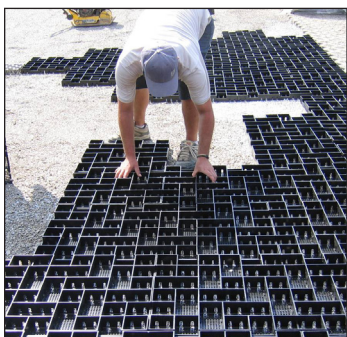
Installing plastic grids over stone.
