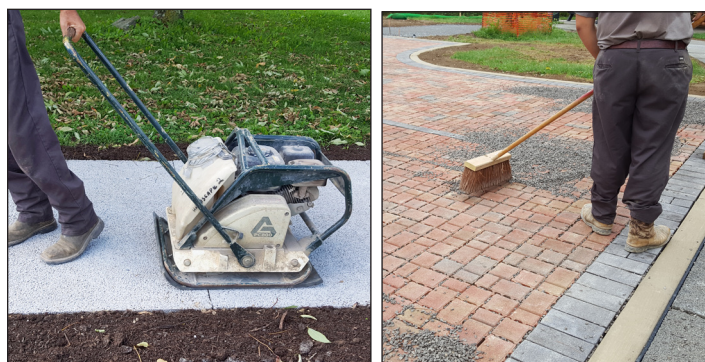
Left - Tamping ; Right - Broom small clean gravel into place.
