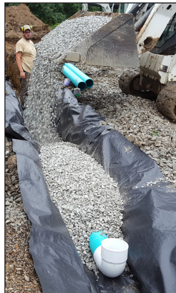
Underdrain being installed with gravel around a perforated pipe. Elbow to receive vertical pipe for future inspections.
