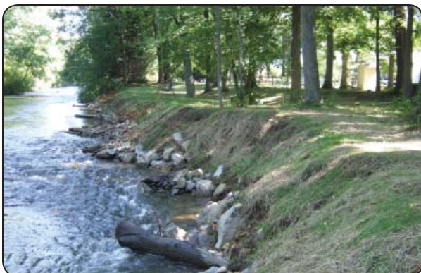
After streambank stabilization
