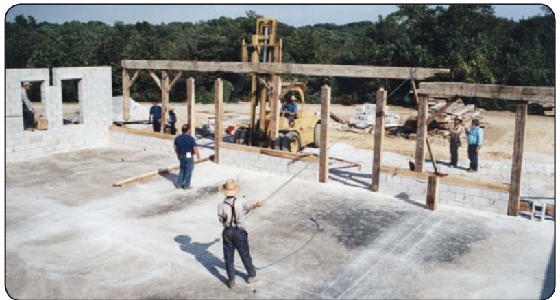
Setting a main beam at the new Donohoe Center location.
