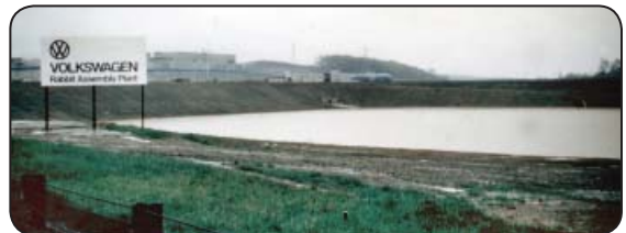
The sediment pond at the Volkswagen plant
