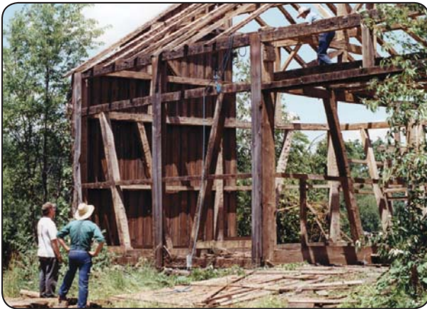
Disassembling the barn in Penn Township.
