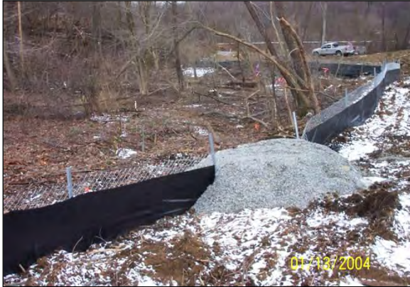
Super Silt Fence with Rock Filter Outlet Photo courtesy of Westmoreland Conservation District
