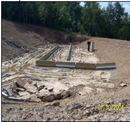
Jersey barrier baffles being used Photo courtesy of Westmoreland Conservation District
