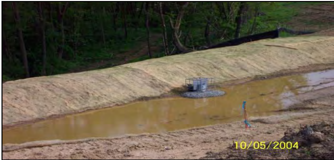
Riser spillway sediment trap Photo courtesy of Westmoreland Conservation District
