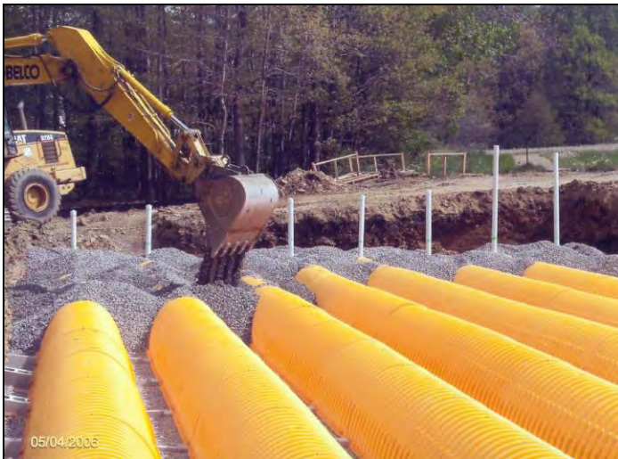
Underground infiltration chamber installation showing cleanouts Photo courtesy of Bove Engineering Inc
