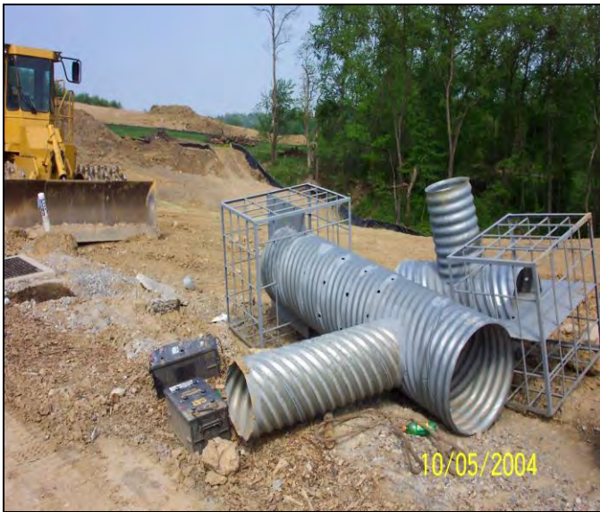
Temporary riser before installation Photo courtesy of Westmoreland Conservation District
