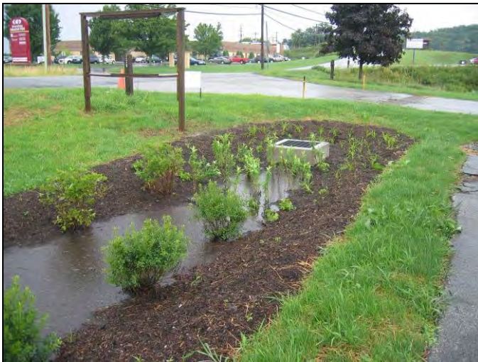
Example of bio-infiltration swale Photo courtesy of Westmoreland Conservation District
