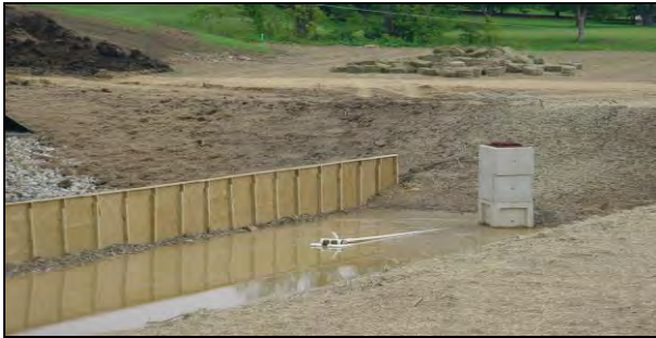
Plywood baffle being used with skimmer dewatering device. Note: Baffle is extended into side of basin Photo courtesy of Westmoreland Conservation District
