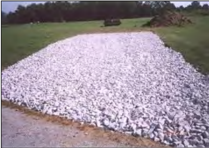
Rock Construction Entrance. Photo courtesy of PaDEP
