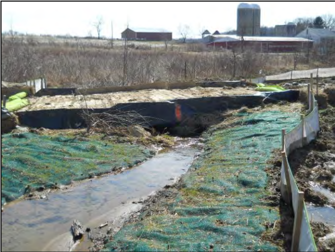
Timber mat wetland crossing Photos courtesy of WCD
