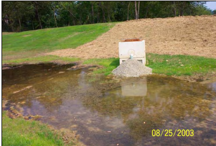
Type M inlet box permanent riser Photo courtesy of Westmoreland Conservation District
