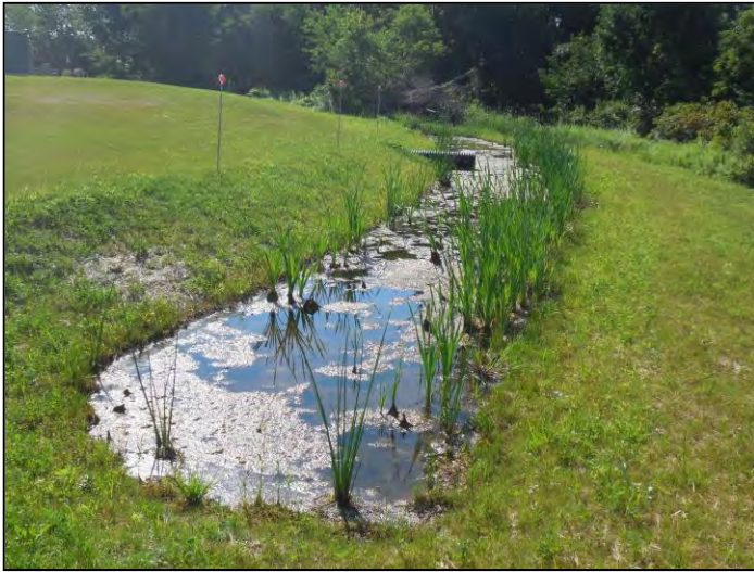
Poorly designed level spreader – constructed level with a stabilized downslope berm, but there is no alternative to drain the system
