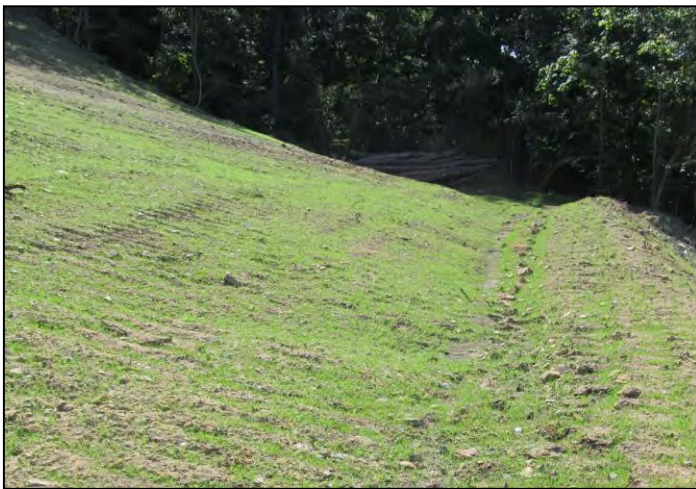
Water Bars on a utility corridor
