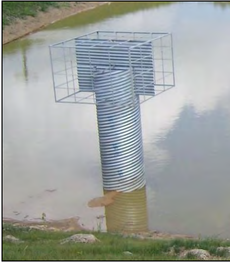
Trash rack and anti-vortex mounted on temporary riser Photo courtesy of Westmoreland Conservation District
