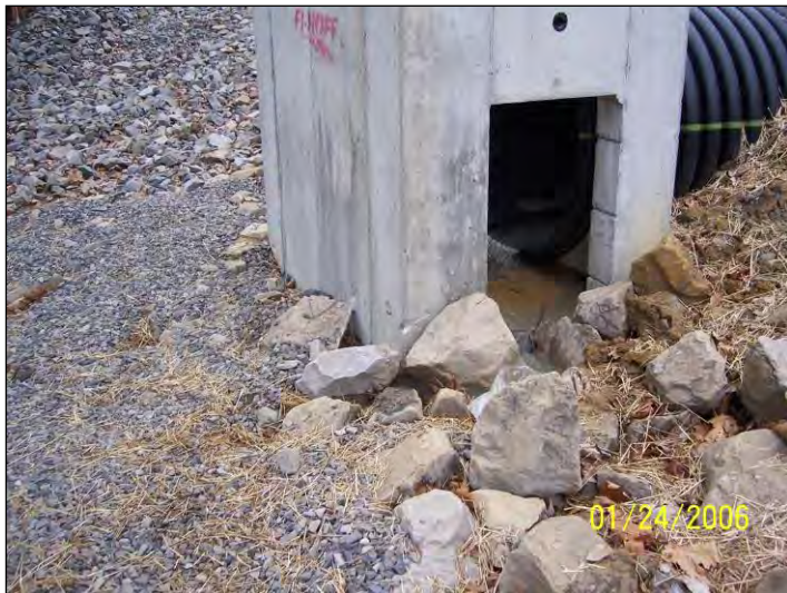
T-Outlet energy dissipater using Type M inlet Photo courtesy of Westmoreland Conservation District
