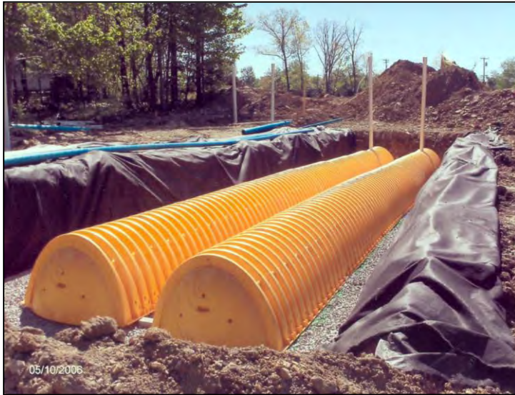
Underground chamber system being installed as a dry well. Photo courtesy of Bove Engineering Inc.
