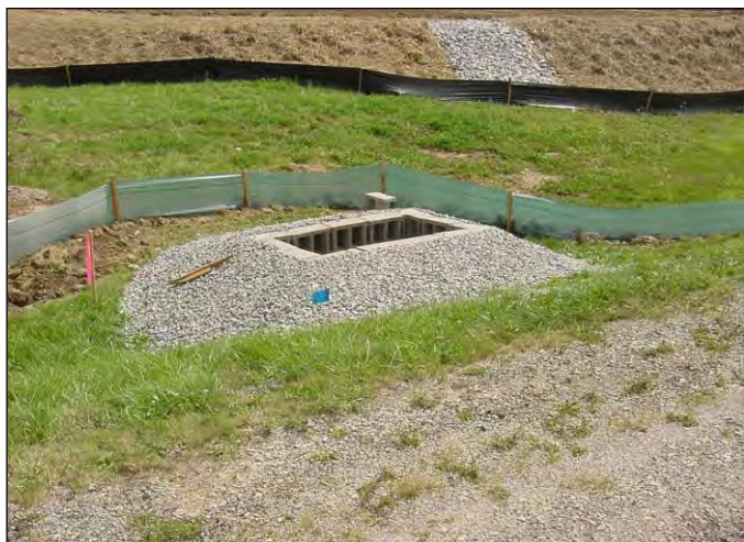
Concrete Block Inlet Protection Photo courtesy of PaDEP
