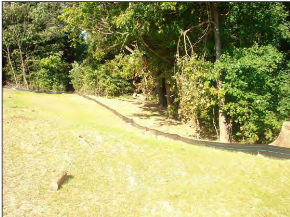
Standard Silt Fence Photo courtesy of PaDEP
