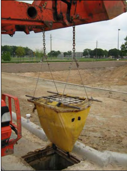
Filter bag inlet protection. Photo courtesy of ACF Environmental.
