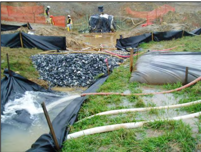
Flume (above) and pump bypass for stream crossing Photos courtesy of WCD and DEP
