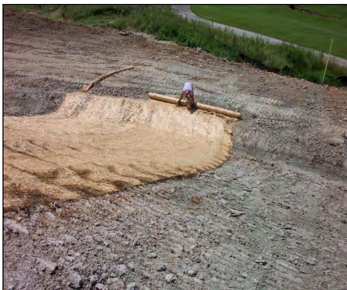
Turf reinforced mat being laid on a slope Photo courtesy of Westmoreland Conservation District
