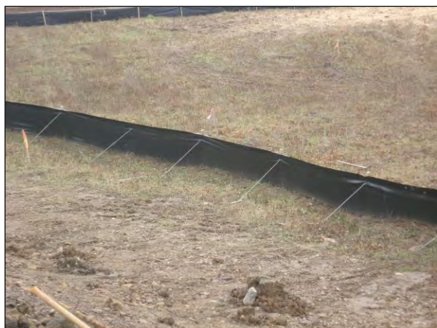
Standard reinforced silt fence Photo courtesy of PaDEP
