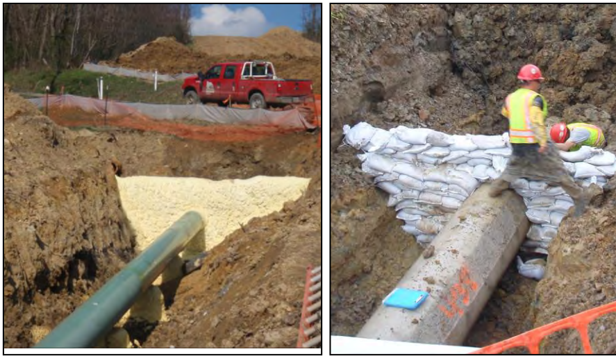
Foam trench plug (left) and sand bag trench plug Photos courtesy of WCD and DEP
