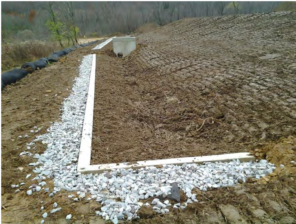
Well-designed level spreader – constructed with t-outlet and stable downslope berm, using concrete curb
