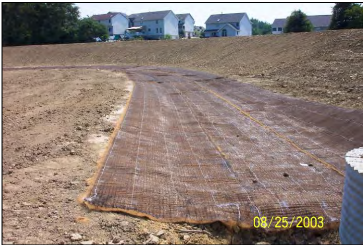
Turf reinforcement mat in a channel Photo courtesy of Westmoreland Conservation District
