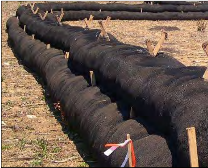
Compost Sock Sediment Trap Photo provided by Filtrex™
