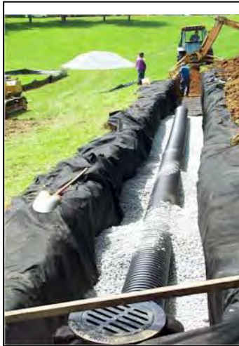
Infiltration trench during and after installation. Photos courtesy of Pa DEP Stormwater Best Management Practices Manual
