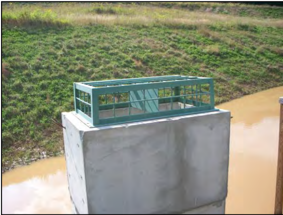
Angle iron and rebar trash rack Photo courtesy of Westmoreland Conservation District
