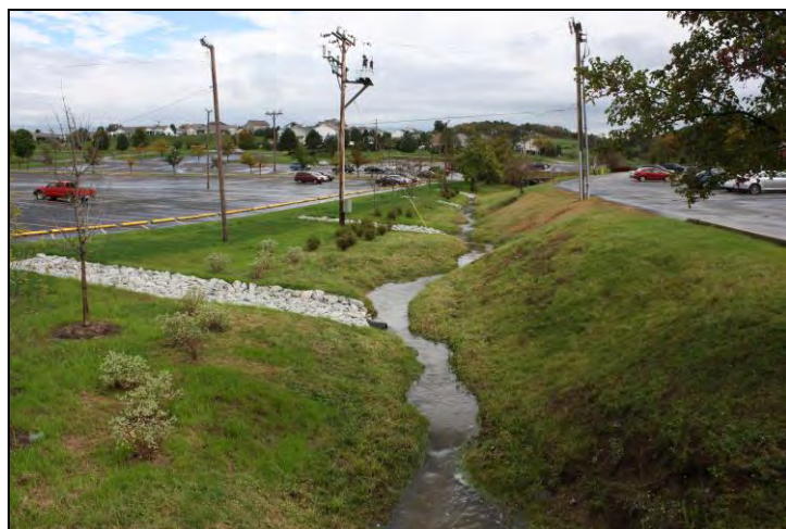
Establishing a riparian buffer along one side of an impacted stream channel, Youngwood PA Photo courtesy of Westmoreland Conservation District
