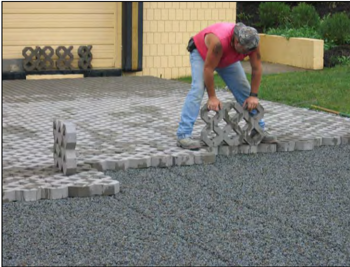
Turfstone™ paving block installation over porous base Photo courtesy of Westmoreland Conservation District
