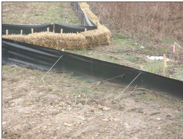
Silt fence with straw bales
