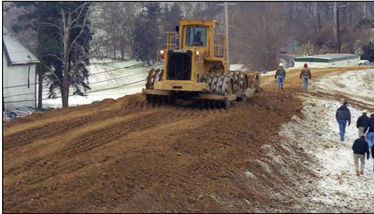
Sheepsfoot roller compacting an embankment Photo courtesy of Westmoreland Conservation District
