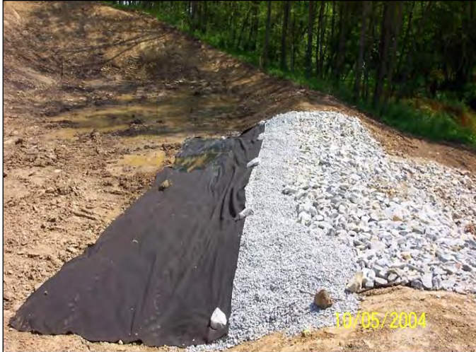
Embankment type sediment trap Photo courtesy of Westmoreland Conservation District
