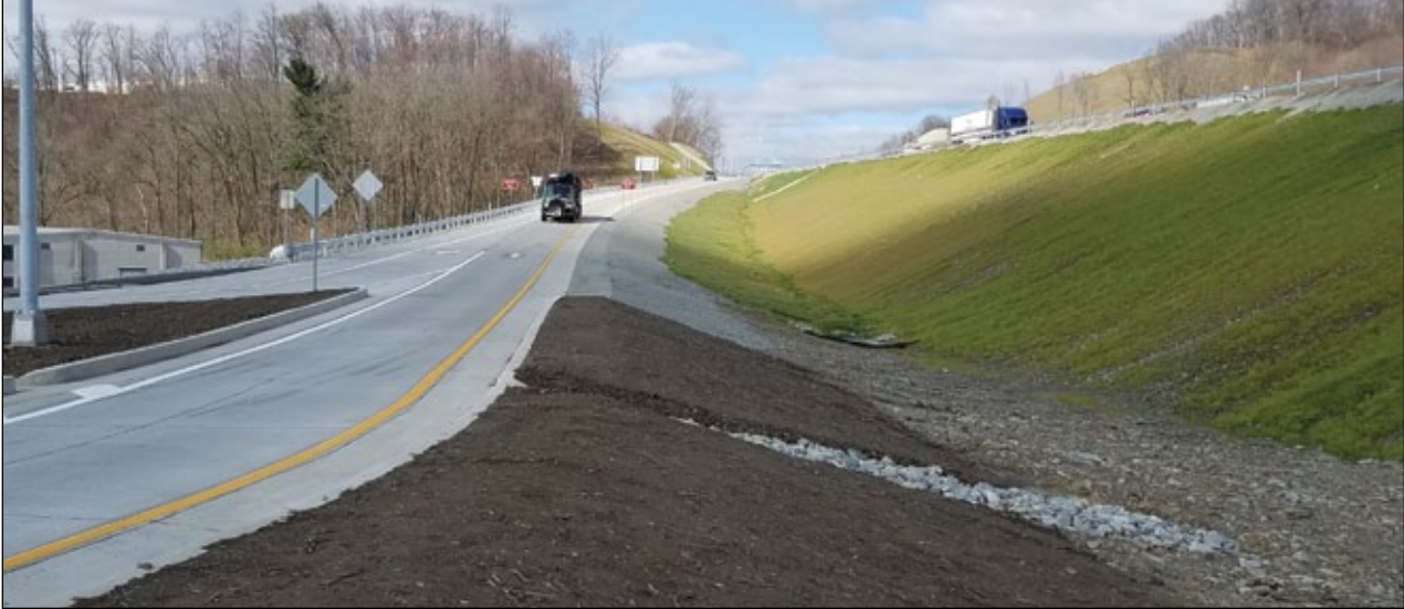
A view of the improved Interstate 70. This eastbound off-ramp at New Stanton was designed so that water from the island (far left), the ramp (center), and the sloped hillside (far right) all will drain into a common infiltration area (low point with rocks). The island and foreground have been dressed with topsoil reclaimed from the site, and will be seeded just as the slope to the far right has been.
