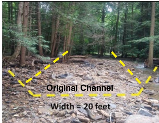
A look at Linn Run upstream from the Valley School shows how rocks and gravel carried by the floodwater completely filled the stream's original channel and forced the water to create an entirely new path (visible on the right side of the photo).
