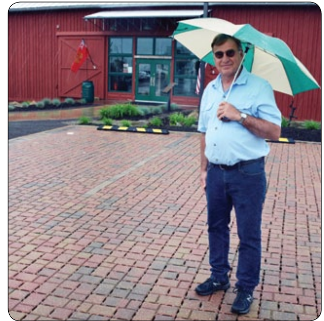
Ron Rohall stands in the parking lot made of permeable pavers, a stormwater management practice, in front of the District headquarters.
