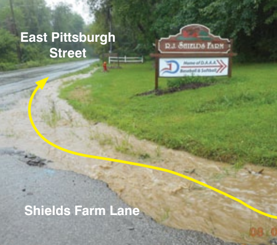
The road to Shields Farm was often plagued with large volumes of stormwater runoff that began at the top of the hilly lane and spilled out onto East Pittsburgh Street, a main street in Delmont.
