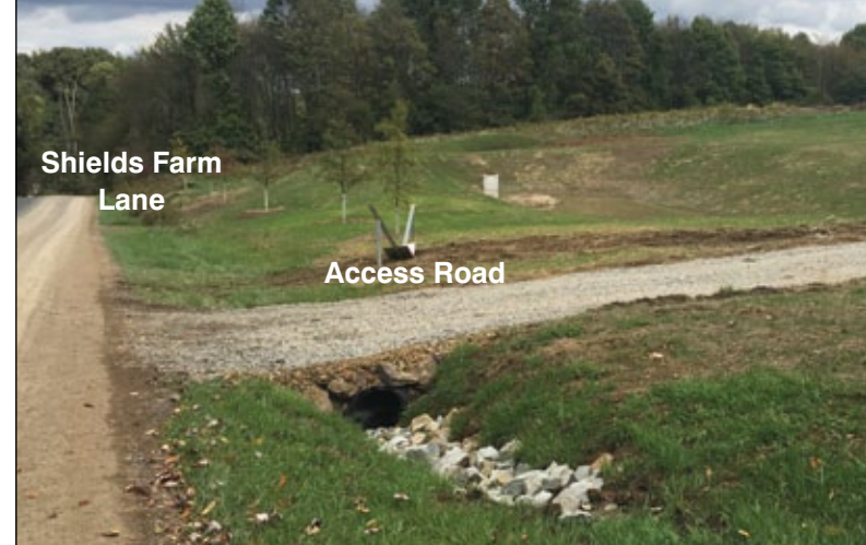
Improvements included a large detention basin (center, background) near the top of the road. Rock riprap and a drainage pipe under an improved access road (foreground) help direct runoff into the new basin.
