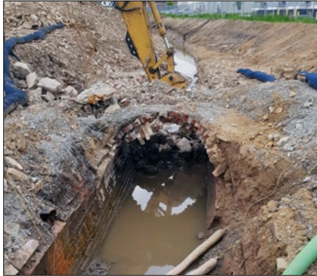
A water course, channeled for decades inside a brick tunnel under six feet of dirt (left photo), was opened up and brought to the surface in a new, 40-foot-wide channel that helps reduce local flooding in Jeannette (right photo).
