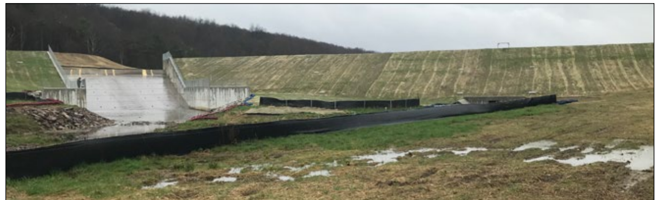
Donegal Lake's new, reconstructed dam and spillway. The long black expanses of cloth are in place to limit the amount of erosion. Grass also was sown at the site to act as another erosion-control measure.
