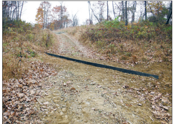
The same section of road with conveyor belt diversions installed
