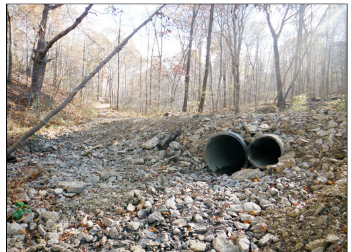
The same crosspipe after being realigned
