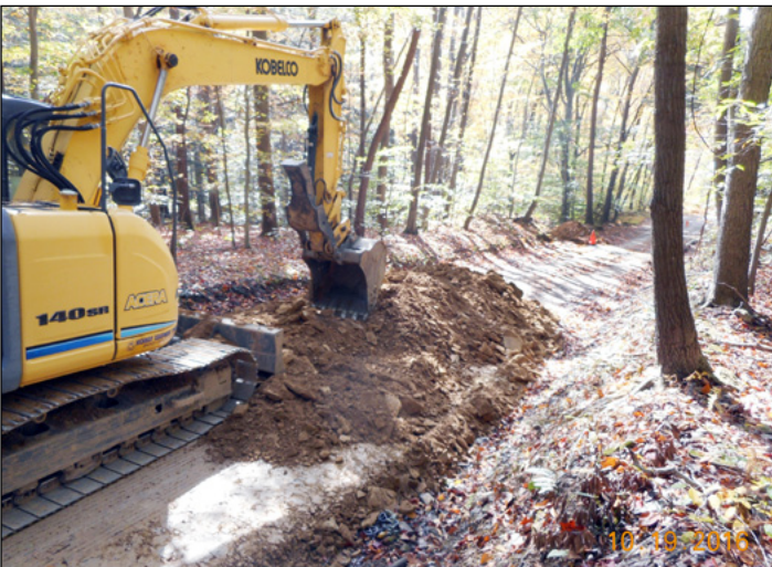
The road profile was filled with shale; Click here for more detailed information on road profiles
