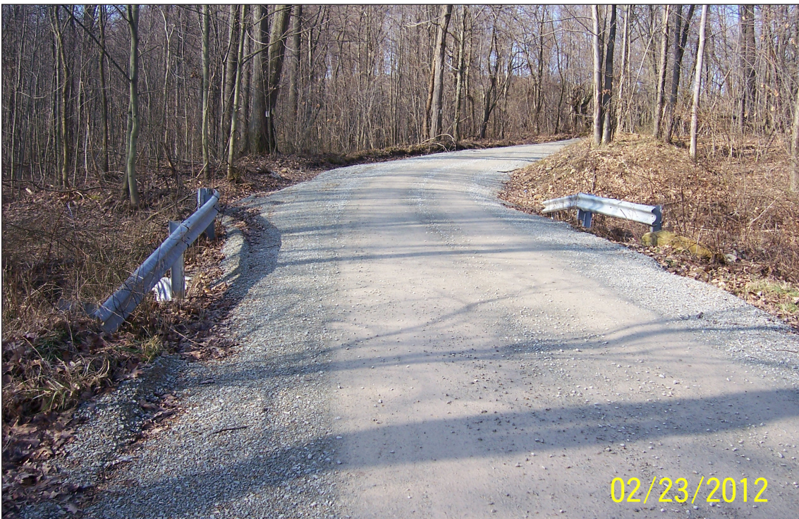
Ridge Road after construction
