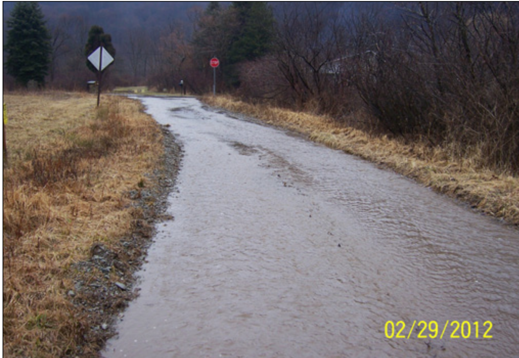
Thomas Road before construction, acting like a stream. Notice the amount of water within the road corridor.
