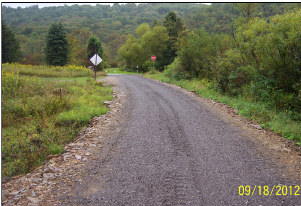
After Construction. Road profile raised 2-3 feet.
