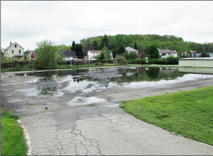
Unused tennis court at the Derry Area Community Pool before construction
