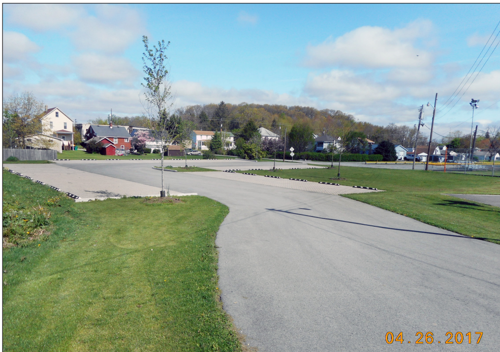
The new parking lot two years after the retrofit
