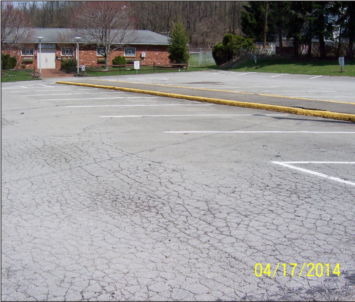
The traffic control island in the parking lot before construction
