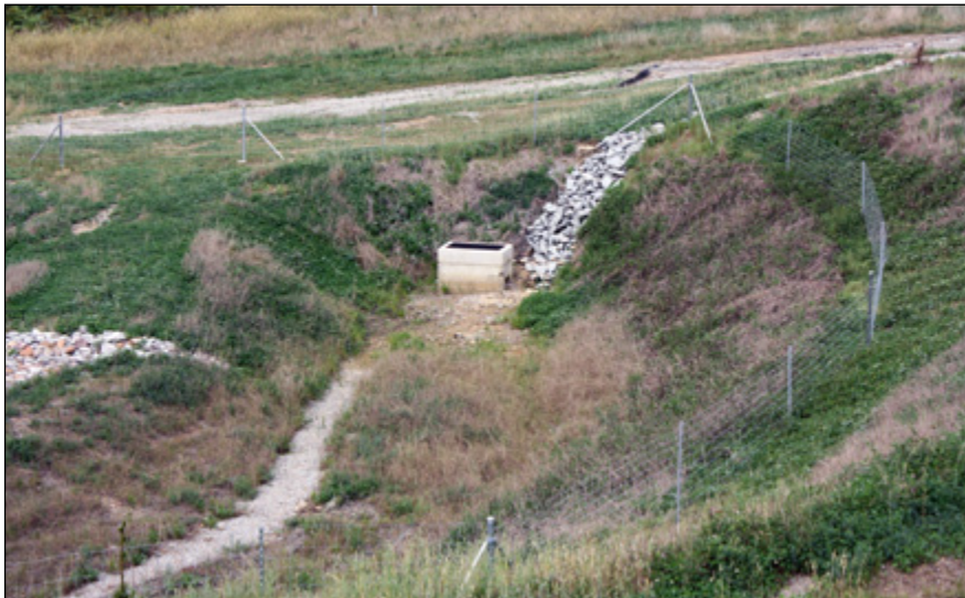
Water quality basin forebay captures the first flush of stormwater runoff and allows the 2 year storm to infiltrate. A 'T-outlet' energy dissipater removes erosive velocity before it enters the forebay.
