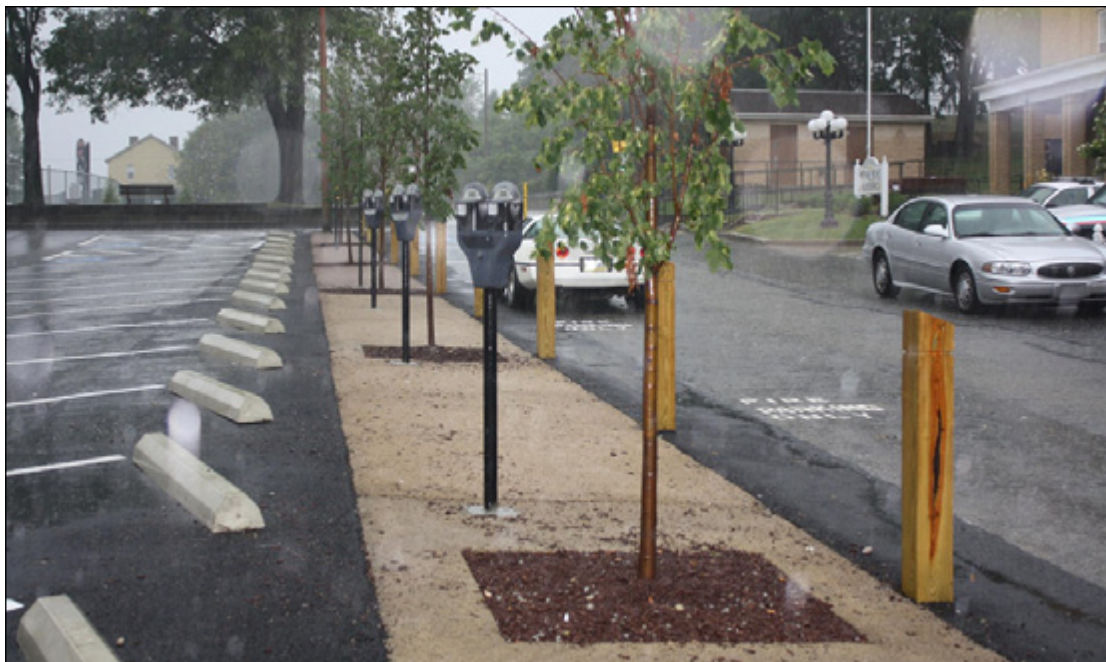
A permeable concrete strip allows stormwater to irrigate newly planted shade trees.
