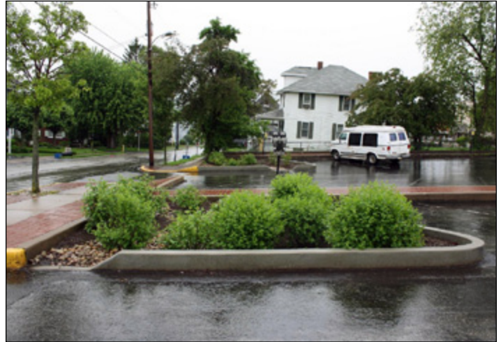
Completed rain gardens capture a portion of parking lot stormwater runoff through curbcuts.
