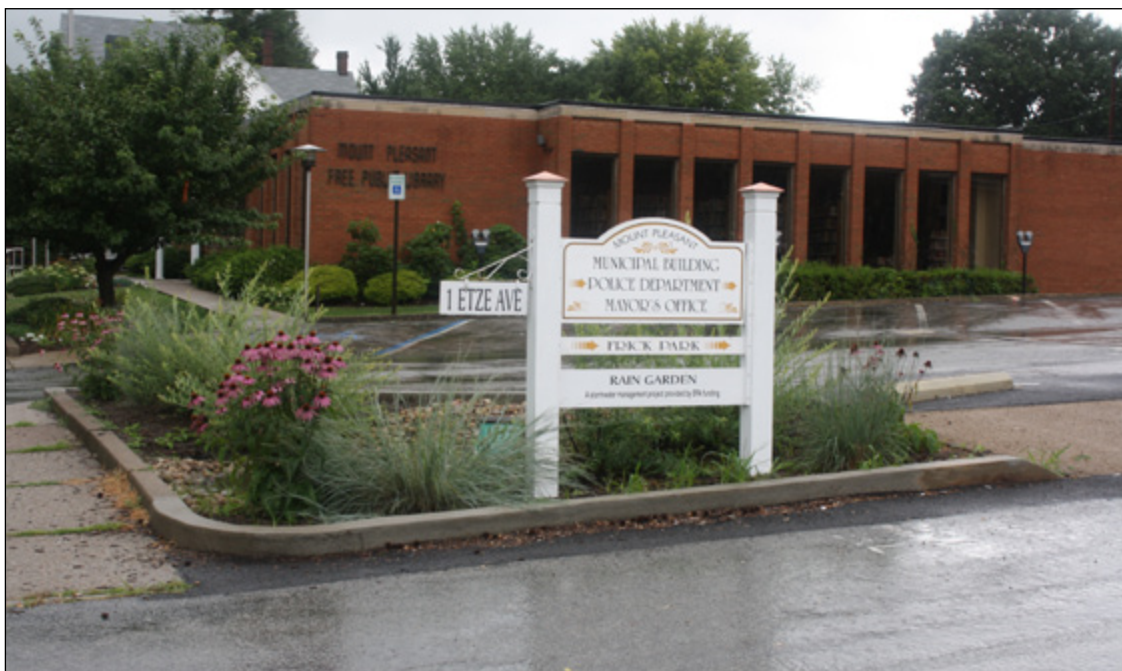
The landscaped rain garden captures and treats a portion of the parking lot stormwater runoff.
