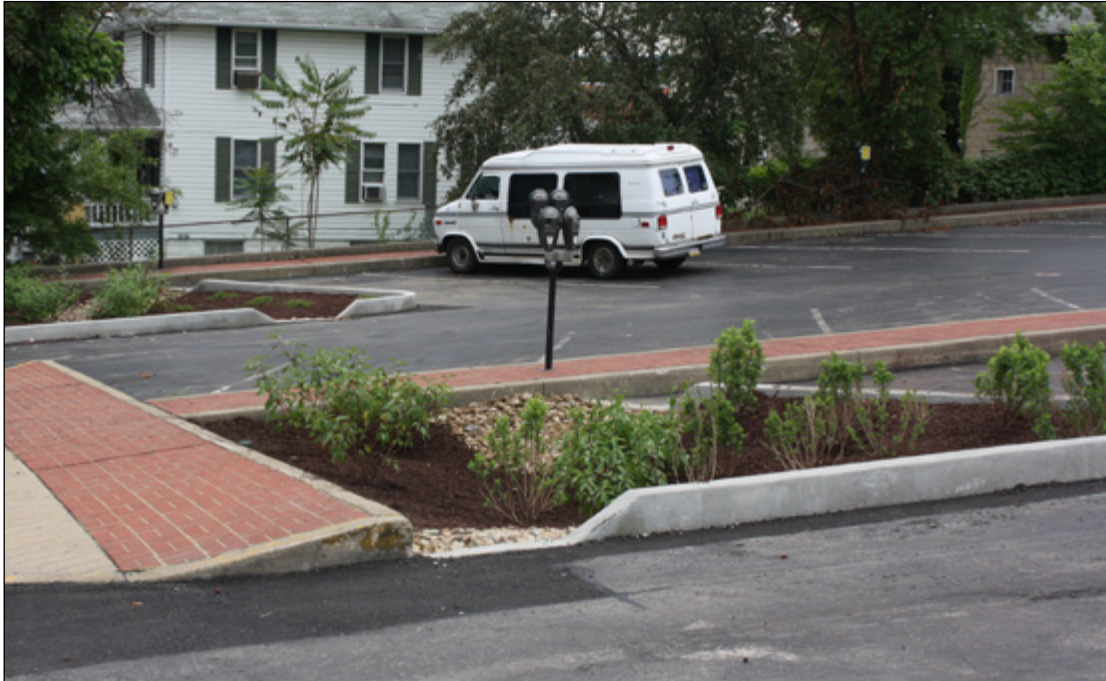
Completed parking lot rain gardens are planted with versatile perennials.
