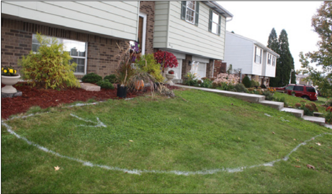
A residential rain garden can be integrated into an existing landscape, but should be at least ten feet from a building foundation
