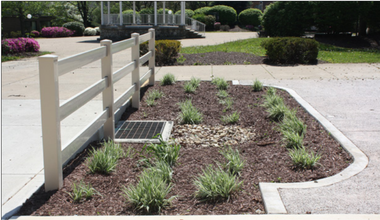
The completed rain garden is landscaped with a grass that can handle versatile conditions.
