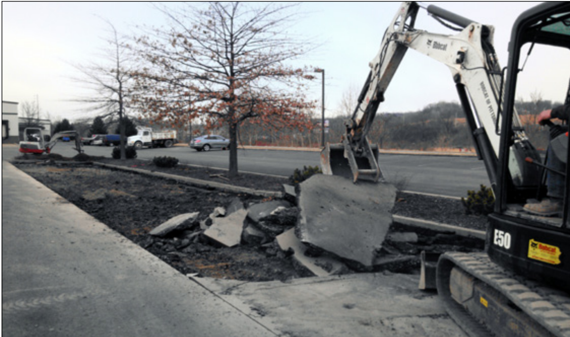
Demolition of existing bituminous paving in existing parking spaces
