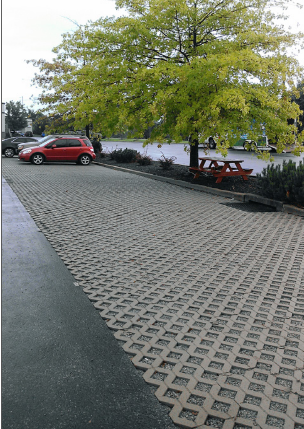
27 parking spaces have been converted to permeable paving.
