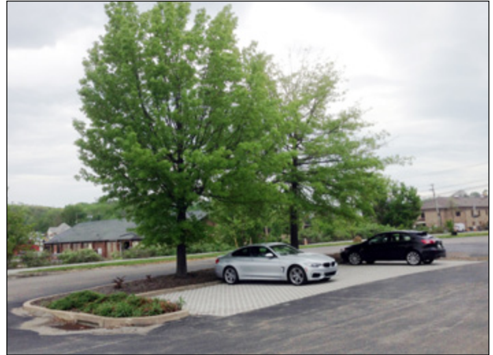
Permeable paving replaces existing asphalt paving to reduce runoff from a parking lot.
