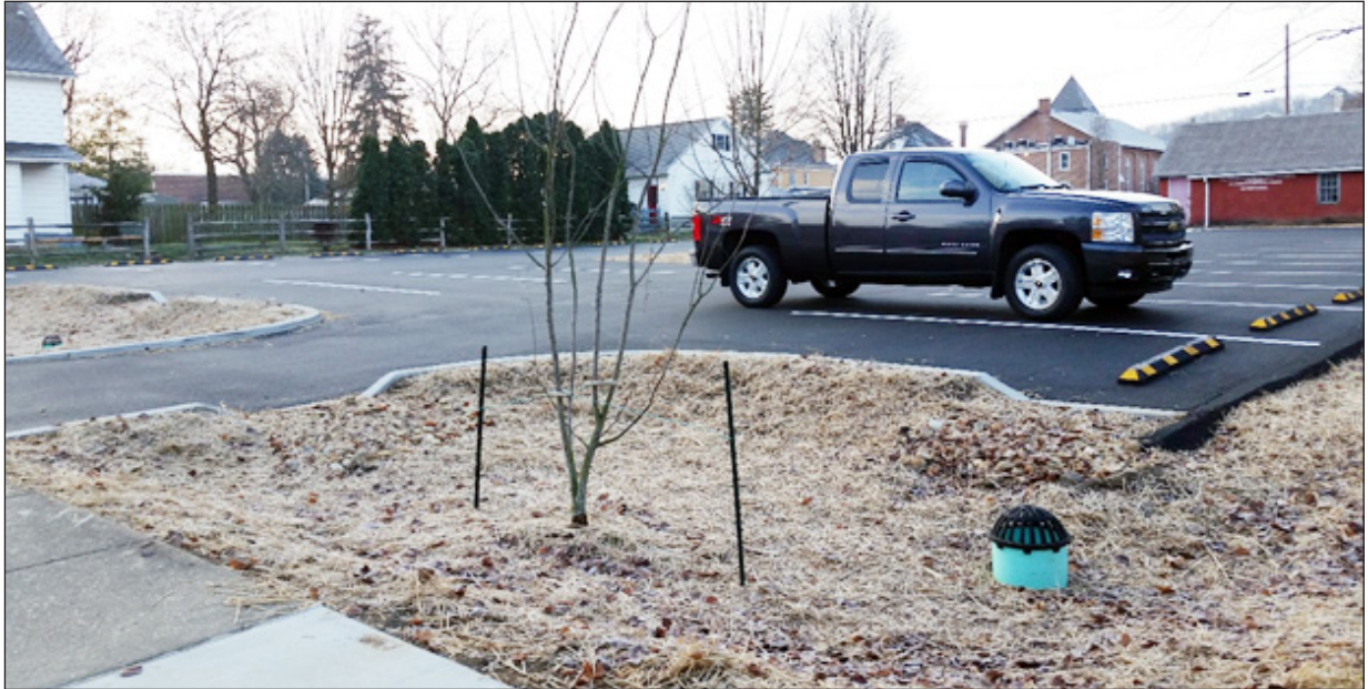
Freshly seeded and mulched, the rain gardens include rock aprons at the curb cuts to slow and spread out the runoff into the rain garden.
