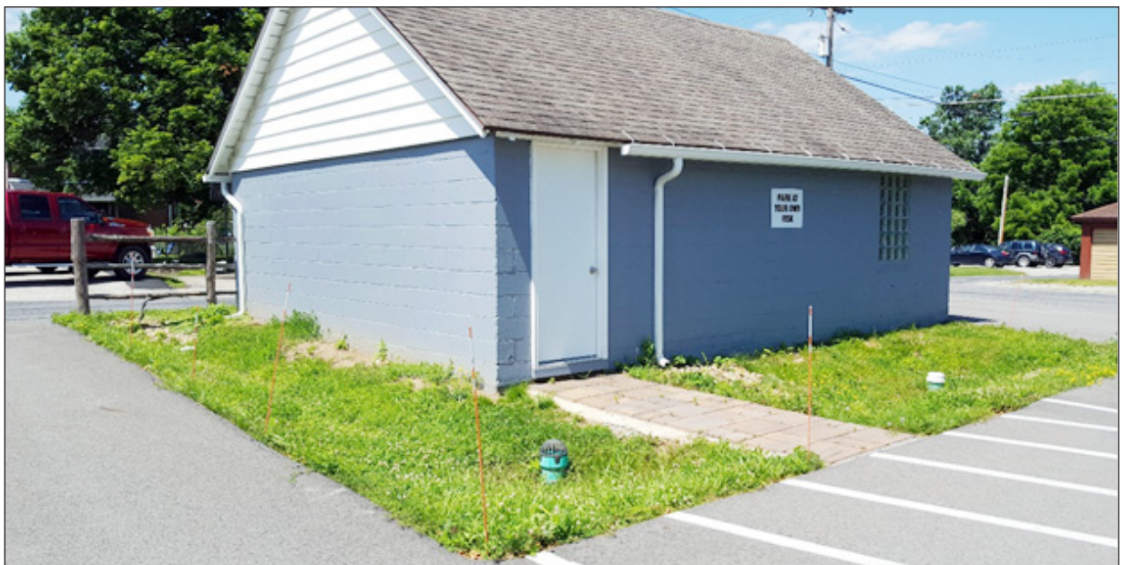
A rain garden, connected by pipe beneath the access path to the storage building, controls a portion of the parking lot as well as the storage building roof runoff. A dense meadow mix covers the surface of the garden.
