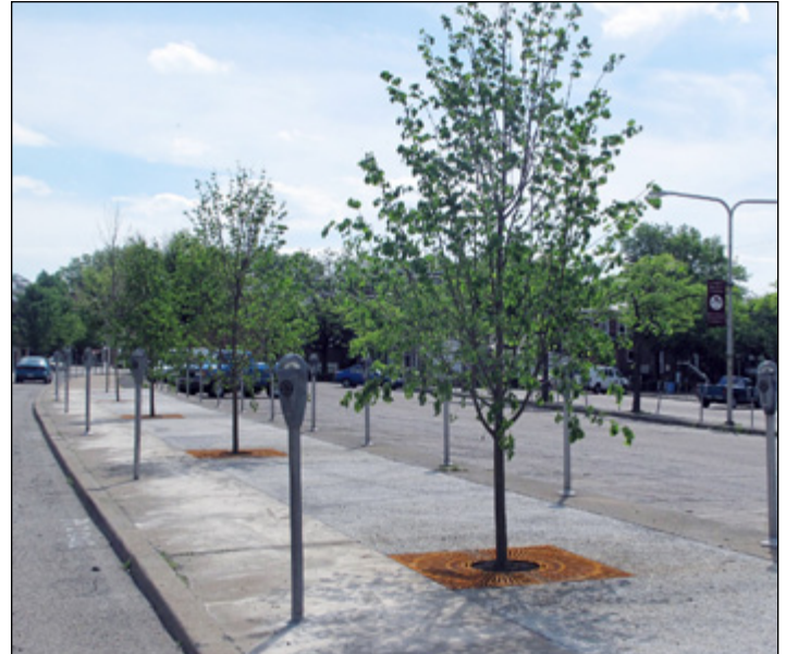
Canopy trees in tree grates over pervious concrete and soil containment system
