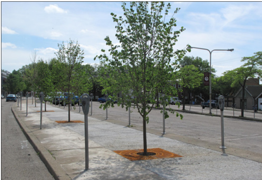
Linden and Sycamore canopy trees in tree grates over pervious concrete and soil containment system
