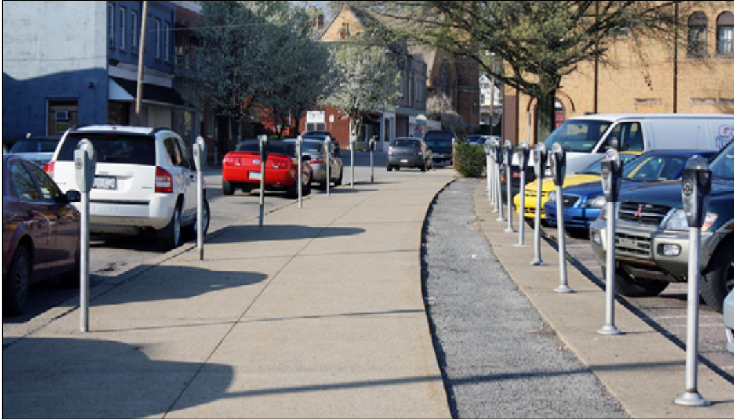
Grant Street sidewalk before project, 16 feet wide sidewalk bordering a Borough parking lot
