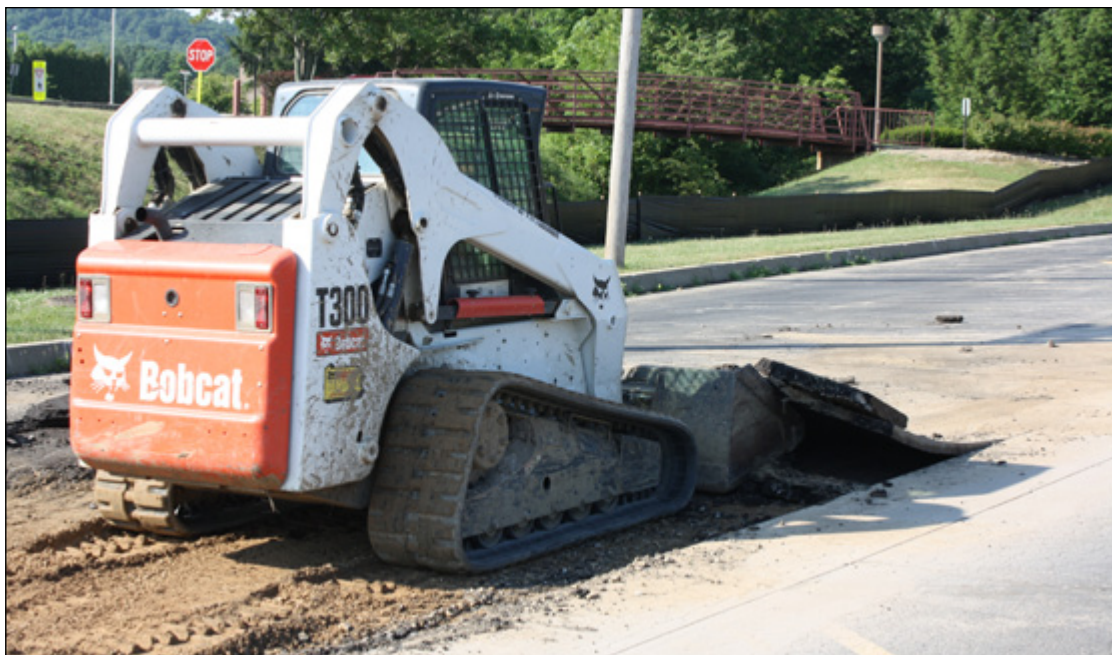
Nearly 1/4 acre of paving was removed to provide a riparian buffer to the stream and to allow for water quality improvements for the stormwater runoff from the parking lot.
