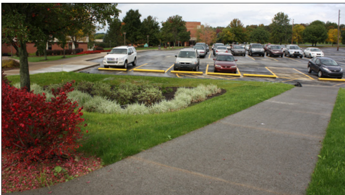
Adjacent to the new permeable concrete walkway is a landscaped rain garden to control a portion of the parking lot stormwater runoff.
