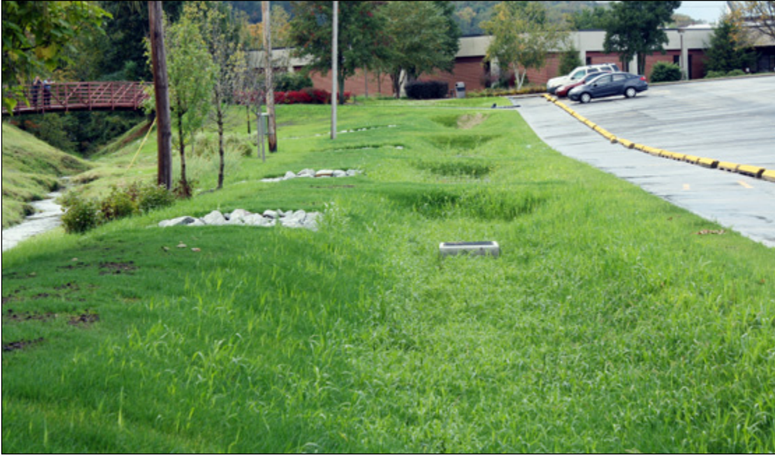
The infiltration trenches were seeded with a vigorous grass mix to promote infiltration and to minimize maintenance.
