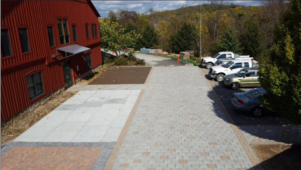
*A combination of seven new and used permeable paving systems are included in the permeable paving demonstration in the rear parking lot at the Westmoreland Conservation District office.*
