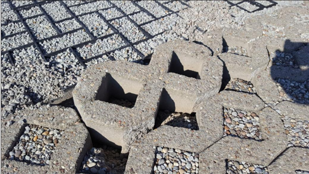
*Existing permeable paving system demonstrations were salvaged for reuse*
