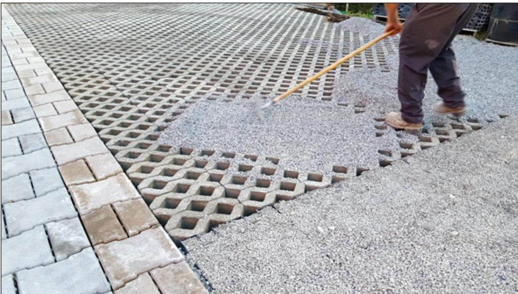
*Number 8 stone is raked into the surface of the salvaged and reused paving systems to continue to provide infiltration in the WCD parking lots.*
