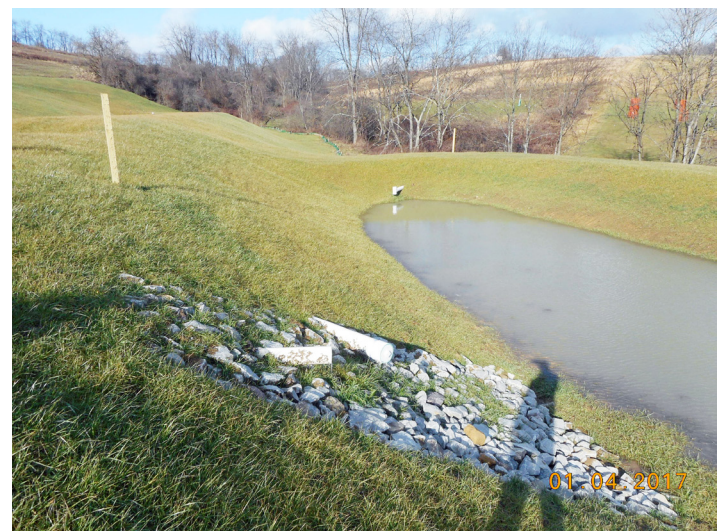
Settling pond 2 about five months after construction
