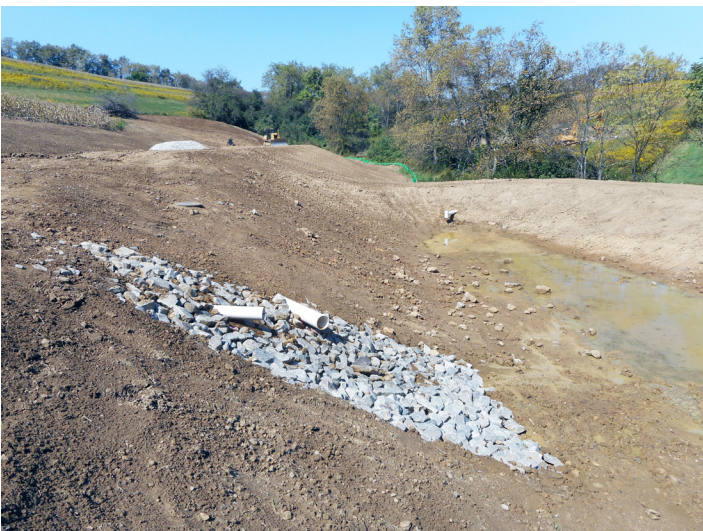
Settling pond 2 directly after construction
