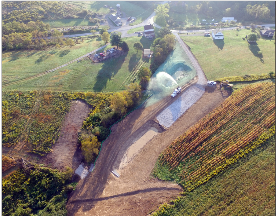
Aerial photo of hydroseeding on finished site
