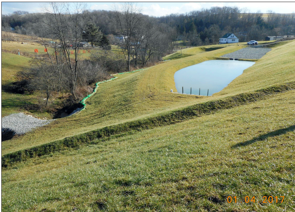
Site after passive treatment system was completed
