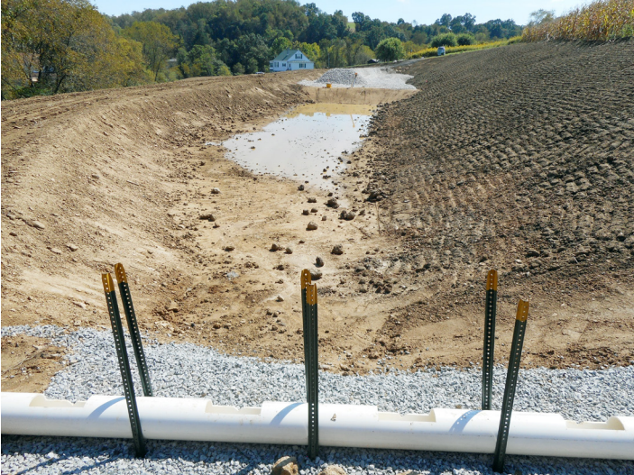
Influent trough and settling pond 1 directly after construction
