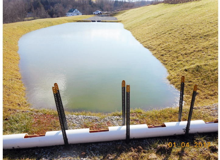
Influent trough and settling pond 1 about five months after construction
