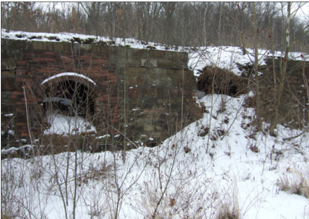
Historic coke ovens adjacent to the Brinkerton Wetland Treatment System.
