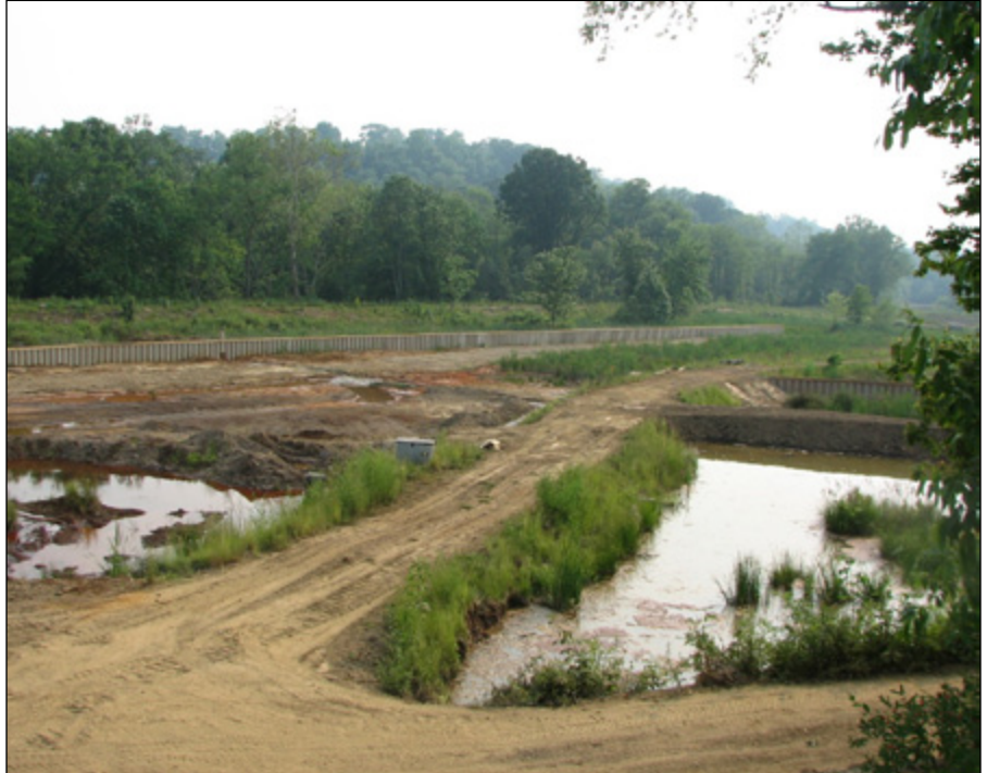
Photo taken during construction of Brinkerton wetland treatment system.
