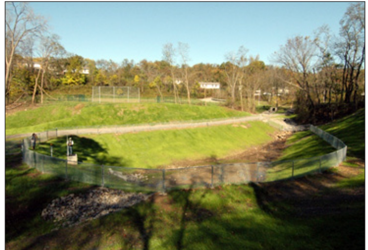
View of completed detention pond project
