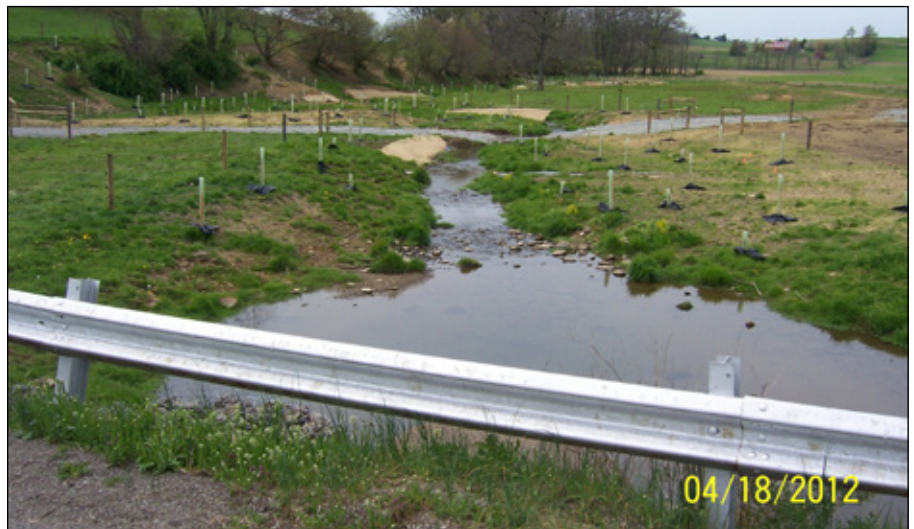
After construction: A stream crossing, stream bank fencing, and riparian buffer was installed to keep the cattle healthier and improve water quality.
