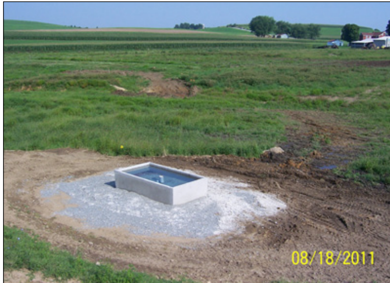
Constructed spring development. This provides cattle with clean spring water instead of muddy creek water.
