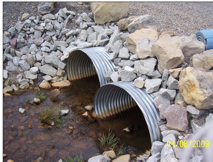
Finished cross pipes carrying Stony Run under a driveway
