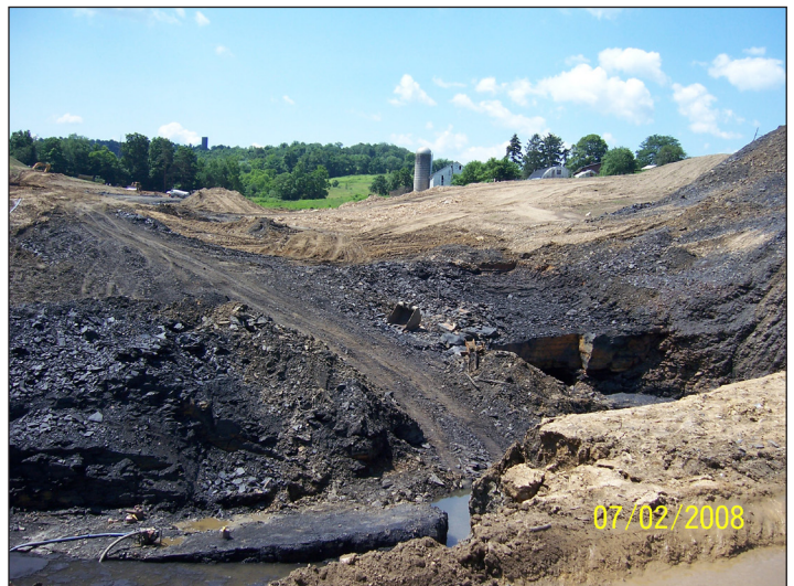
Re-mining in process at the sinkhole before sealing
