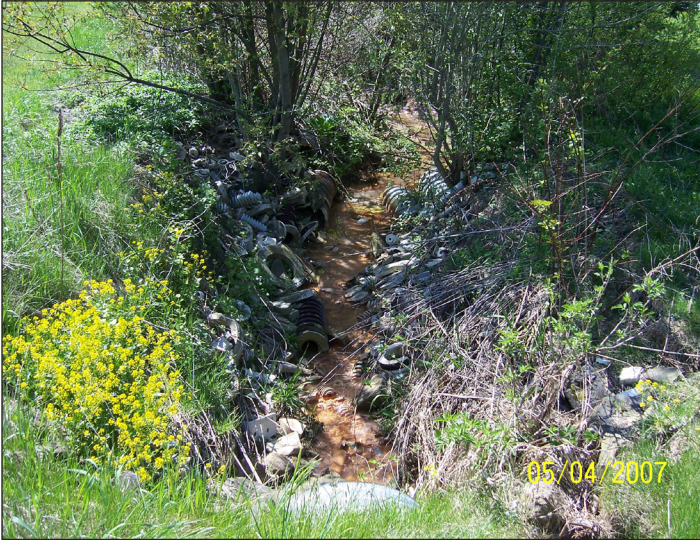
Old cross pipe and streambed before restoration began
