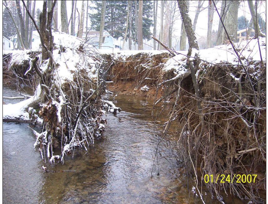
Serious erosion along the bank of Mill Creek at Hannas Run
