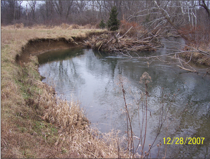
Denison Investment property before any streambank stabilization was done
