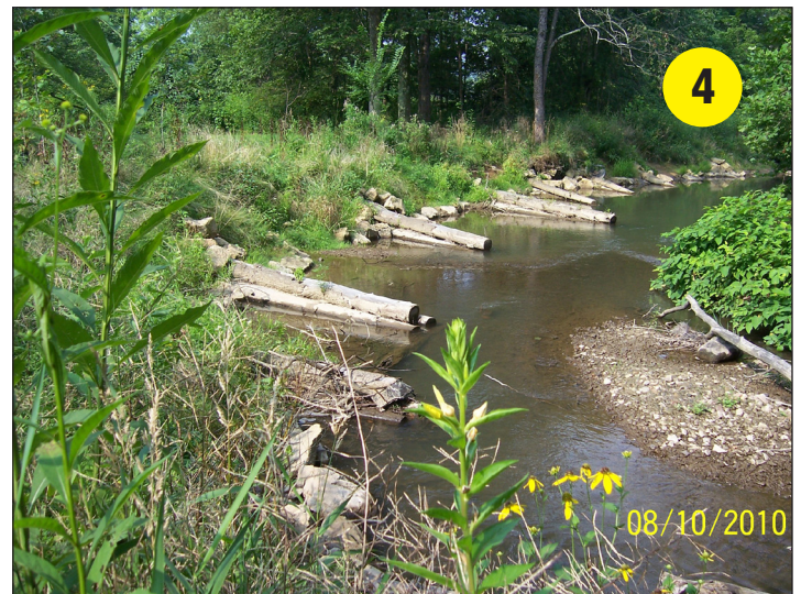
The same streambank two years after construction
