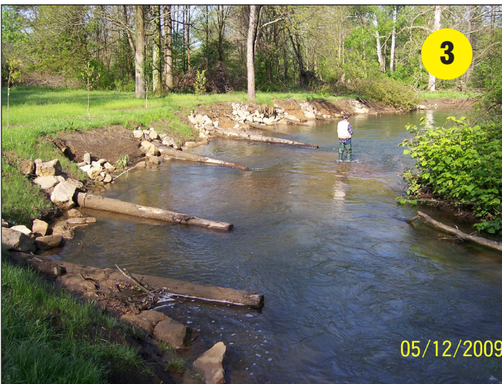
The same streambank almost one year after construction
