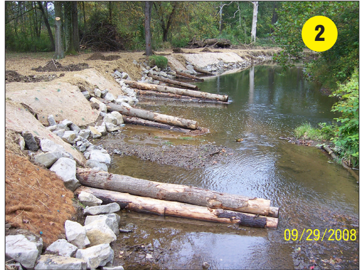
Multi-log vane deflectors installed at the Denison property with rip-rap stabilization
