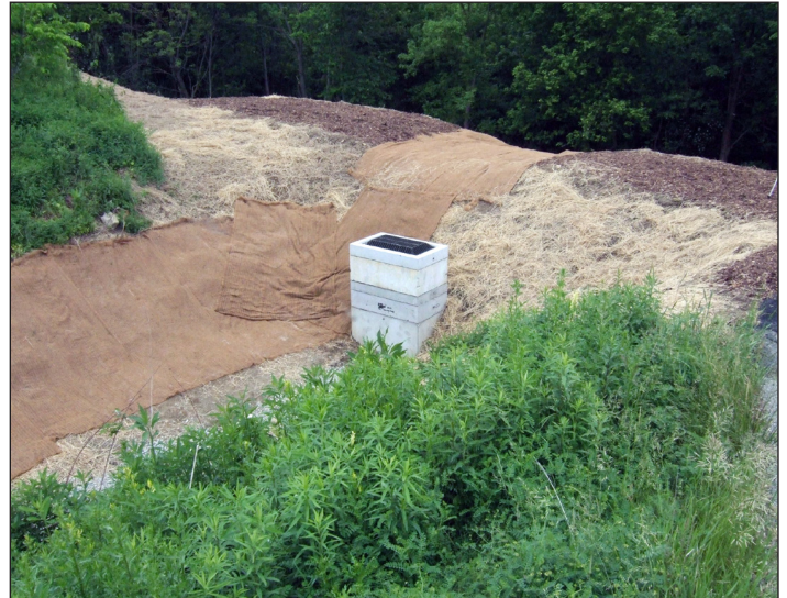
Completed construction of the basin
