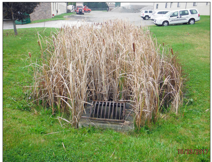
Forebay 10 years after construction
