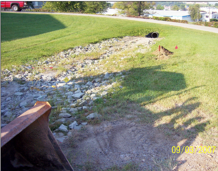
Forebay area of the Bureau of Parks basin before construction
