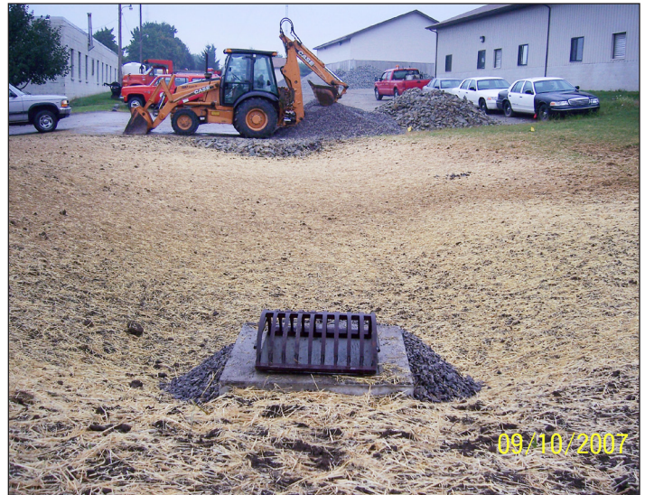
Forebay area after construction
