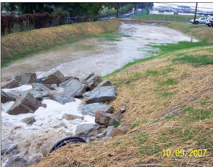
Retention basin at work after a rainstorm
