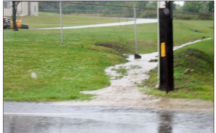
Unmanaged stormwater runoff from the Bureau of Parks and Recreation site before construction flowing onto Donohue Road
