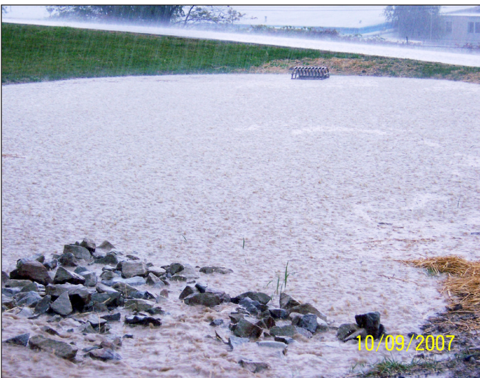
Forebay area managing a rainfall about a month after construction
