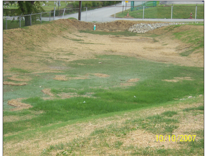
New stormwater retention basin constructed to control stormwater
