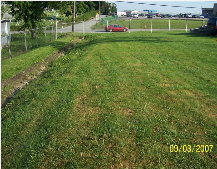
Area by the Bureau of Parks building before main retention pond is installed; uncontrolled stormwater flow directly onto Donohue Road
