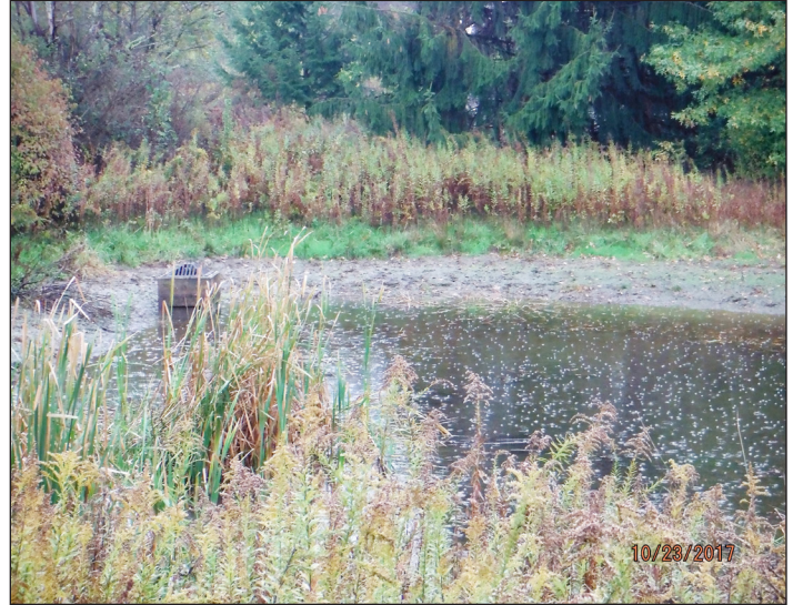
The Donohue basin eight years after retrofitting
