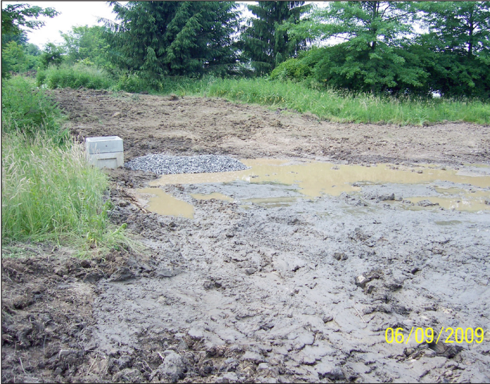
The Donohue basin with a new inlet riser installed
