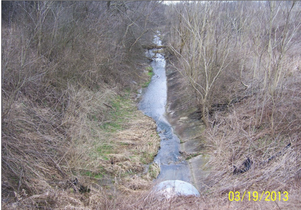
Sherrick Run before mitigation; note the concrete channel lining
