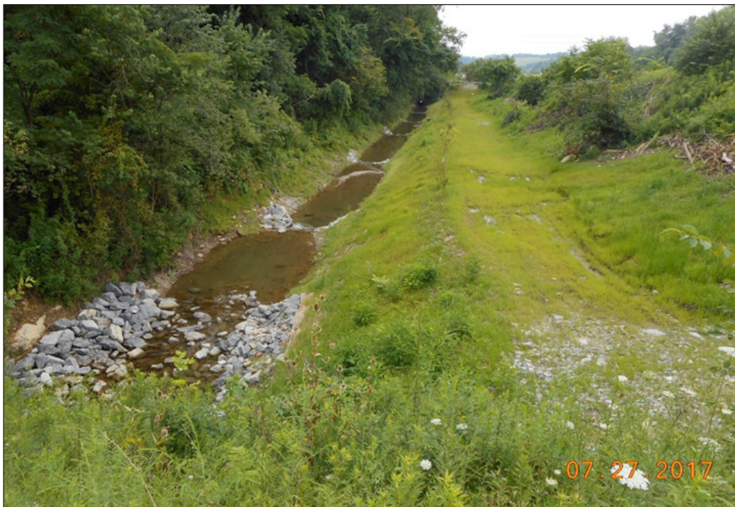
Sherrick Run after mitigation; there is now a natural stream bed and riparian buffer plantings along the banks
