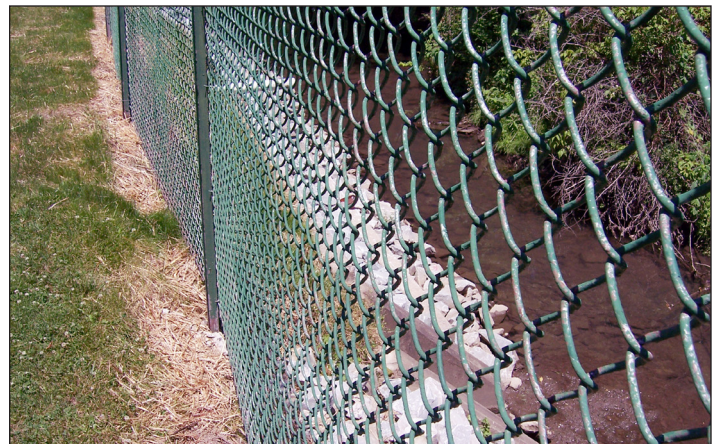
Stabilized bank under fence after rip-rap and riparian buffer planting
