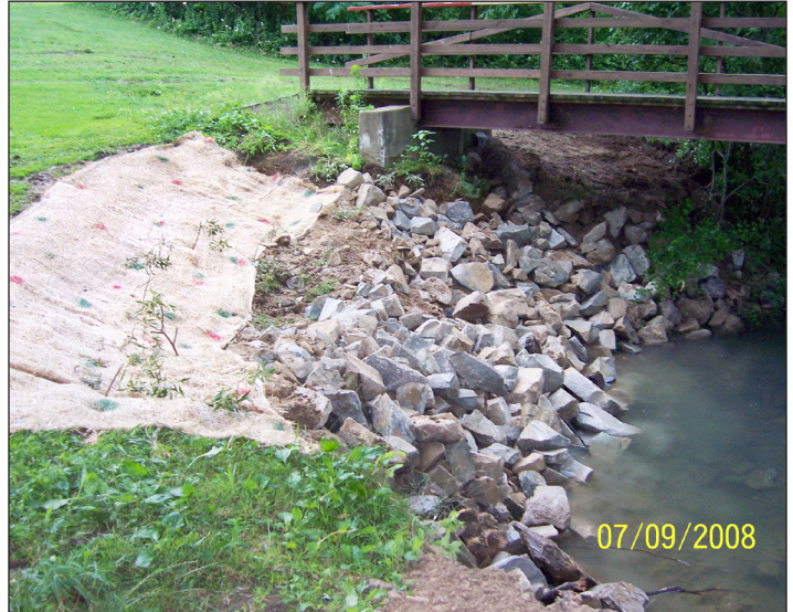
Bank shortly after grading, rip-rap, and seed and mulch
