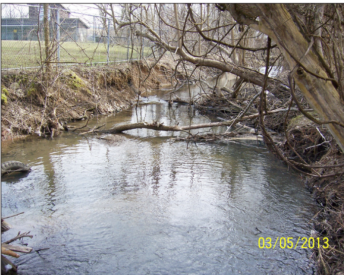
Another Phase II streambank section before construction
