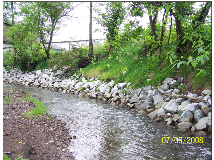
Streambank a few months after construction
