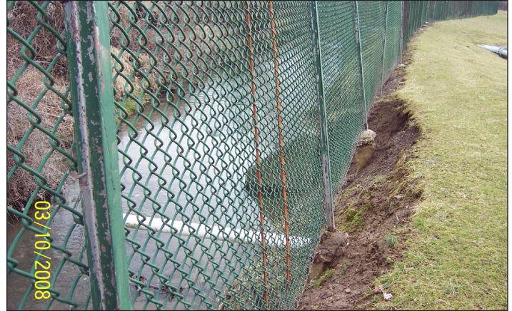
Severe erosion threatening the soccer fields' fence next to Shupe Run
