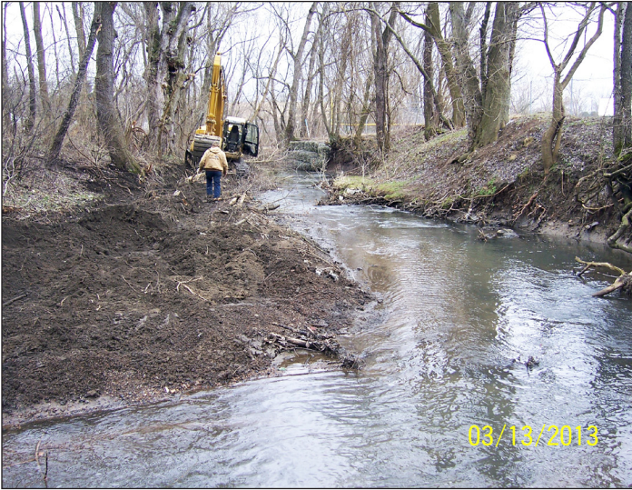
A section of Phase II streambank before construction
