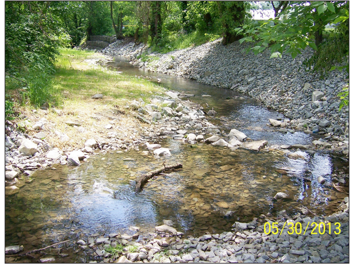
Phase II streambank after construction
