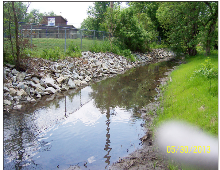
The same section after construction
