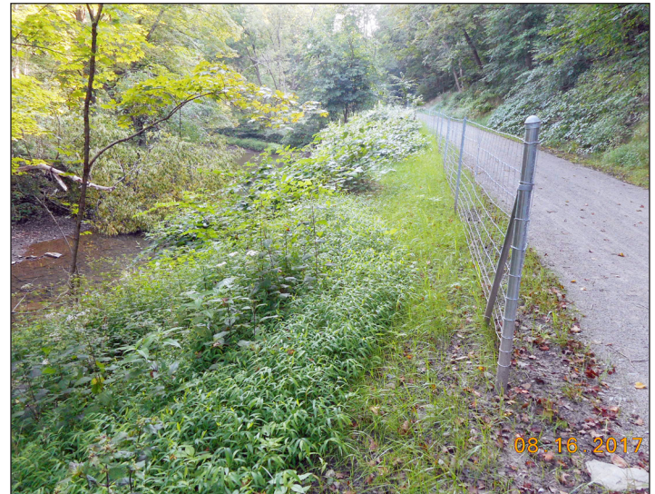
Same section three years after stabilization
