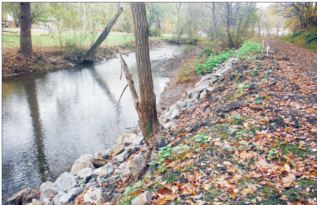
The same tree after the bank was stabilized
