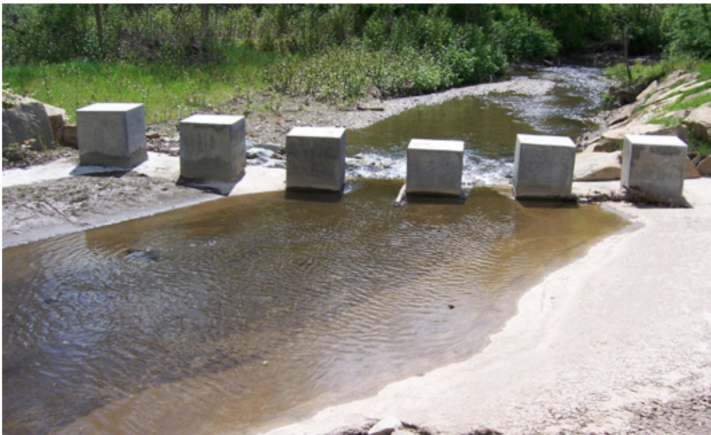
Debris Catcher is designed to trap large debris from continuing downstream and divert it into the debris basin.
