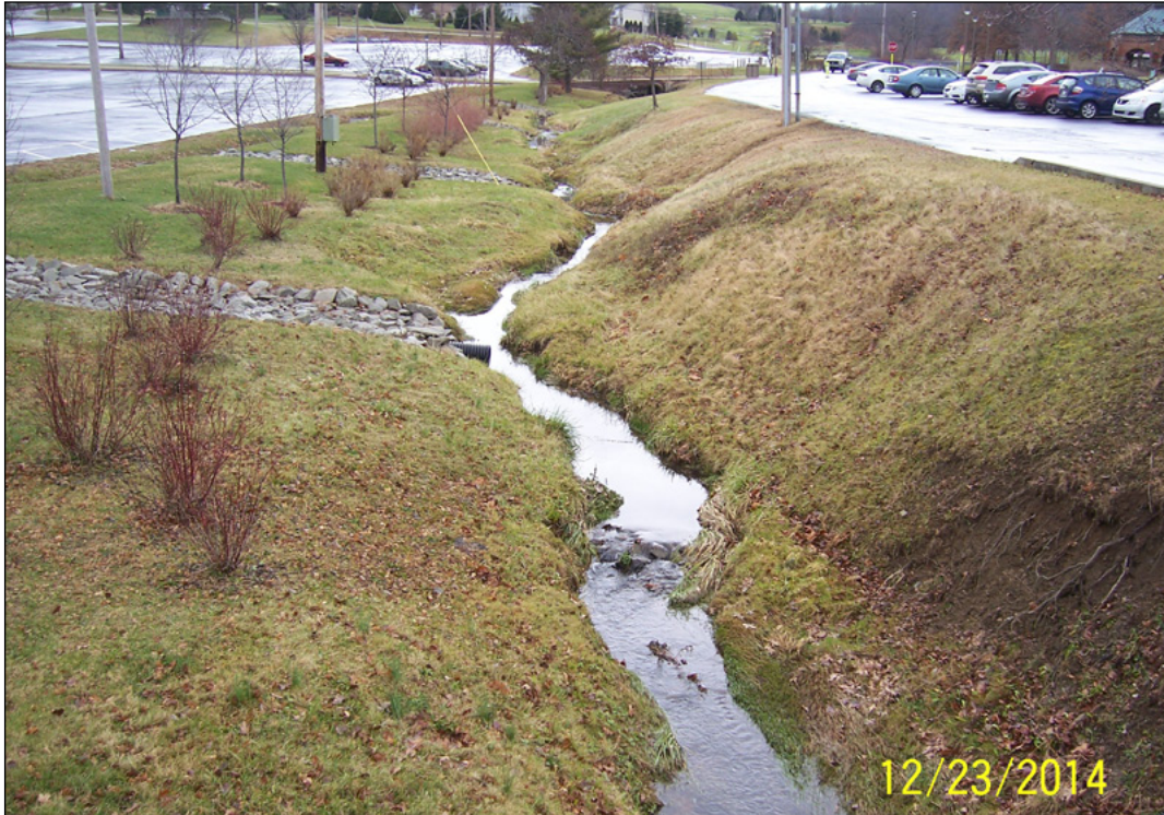
The furthest downstream section of Cherry Creek before construction
