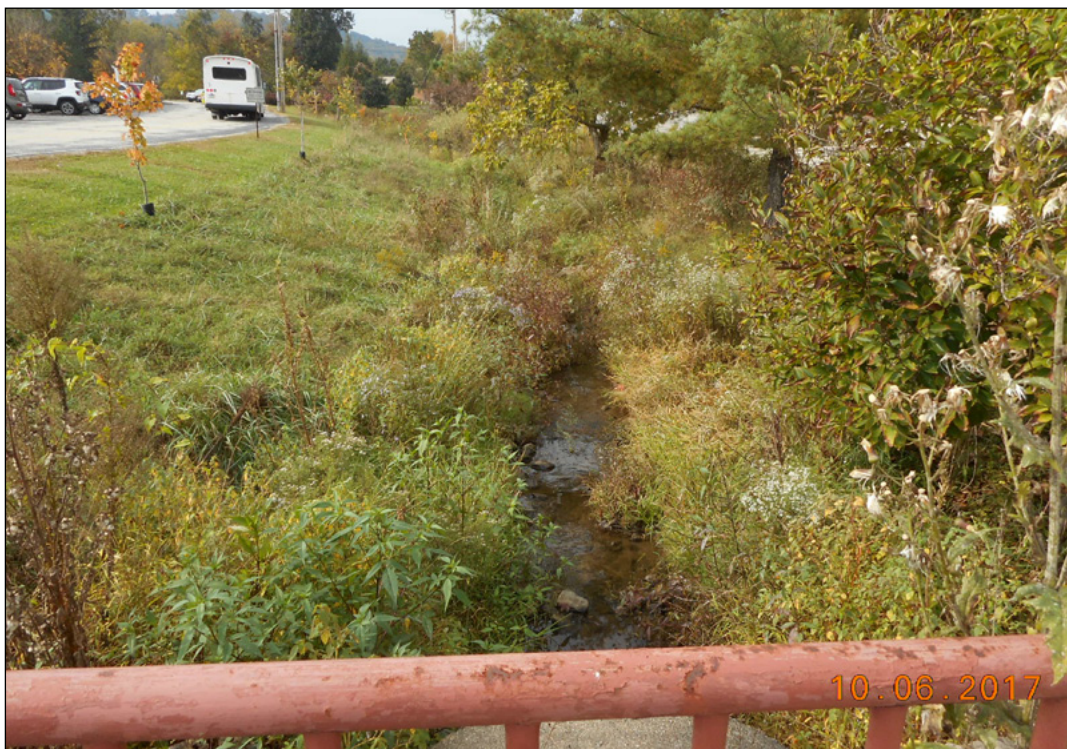
The same section one year after construction
