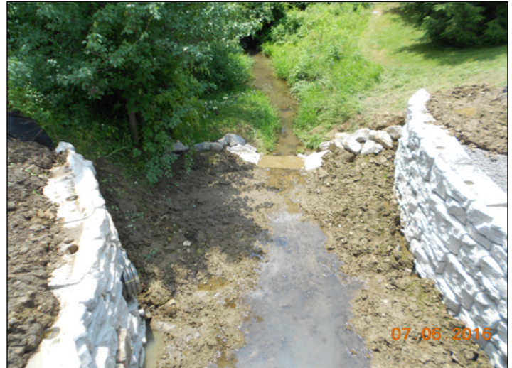
Newly installed Redi Rock walls and rock cross vane
