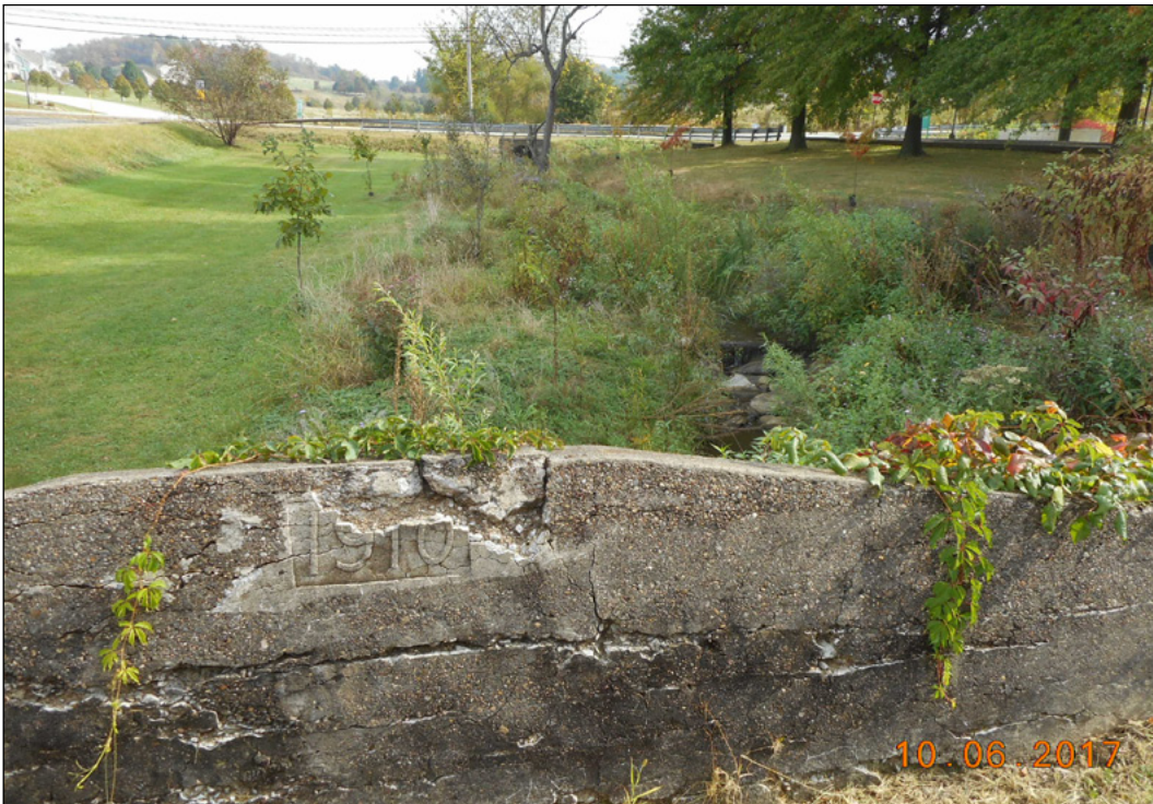
The furthest upstream section a year after construction
