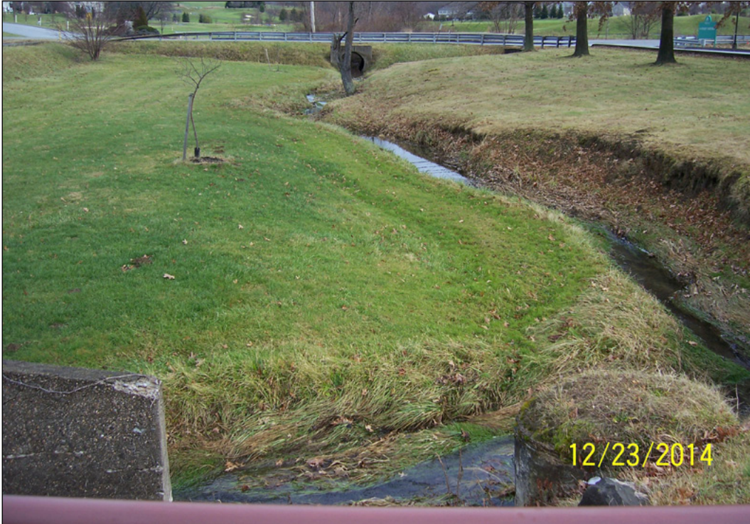
Furthest upstream portion of Cherry Creek before construction; note the mowed banks all the way up to the edge and erosion on the right-hand bank
