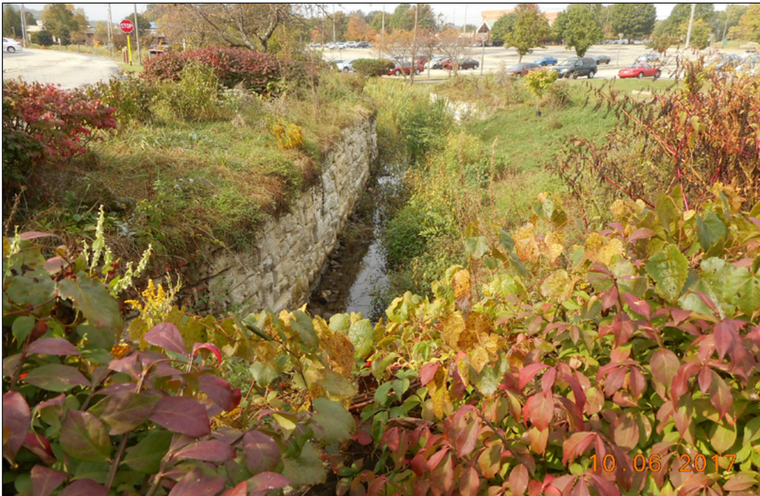
The same section a year after construction with Redi Rock installed in place of the gabion baskets
