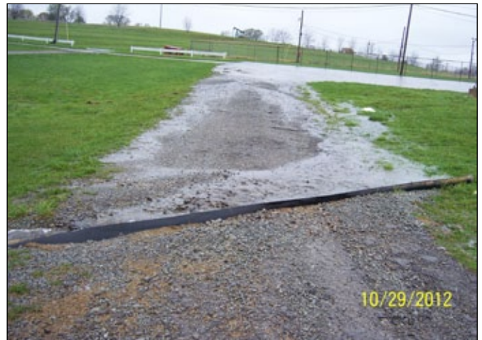
Conveyor belt diversion installed to direct water off of road surface.
