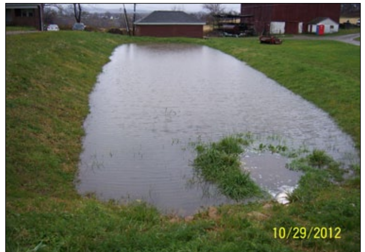
Retention basin managing stormwater after Hurricane Sandy.
