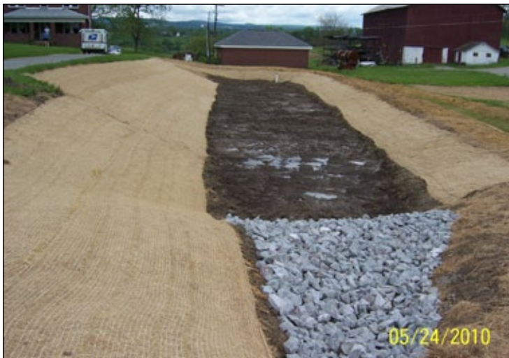
During construction of the retention basin.
