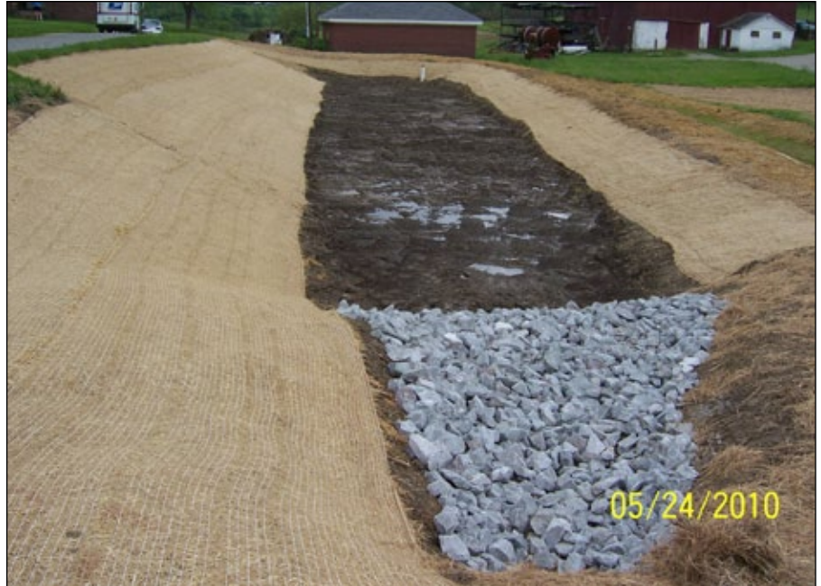
During construction of retention basin.
