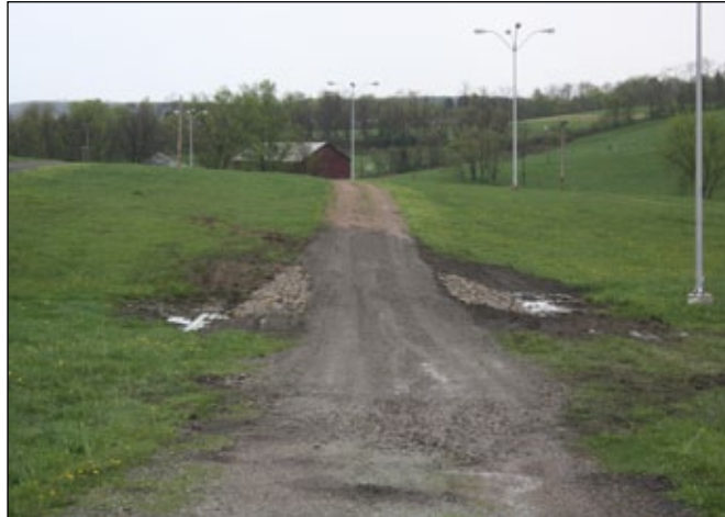
Installation of a French mattress.
