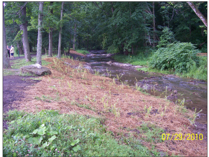
Section of Chartiers Run after construction and riparian buffer planting
