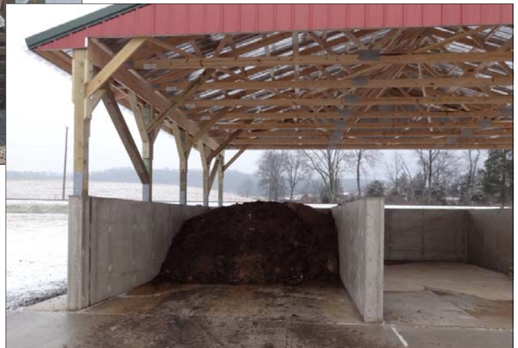
Stand alone poultry mortality composters constructed with treated lumber (left) and concrete walls (below).
