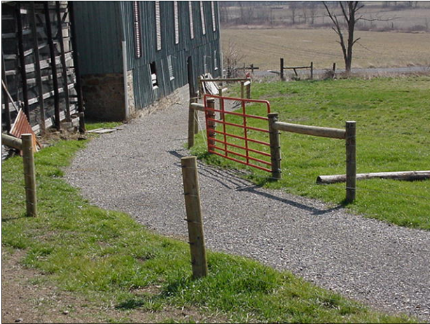
Example cattle walkways at two separate farms (above and left). Geotextile may be needed at some places due to soil type and the nearness to streams.
