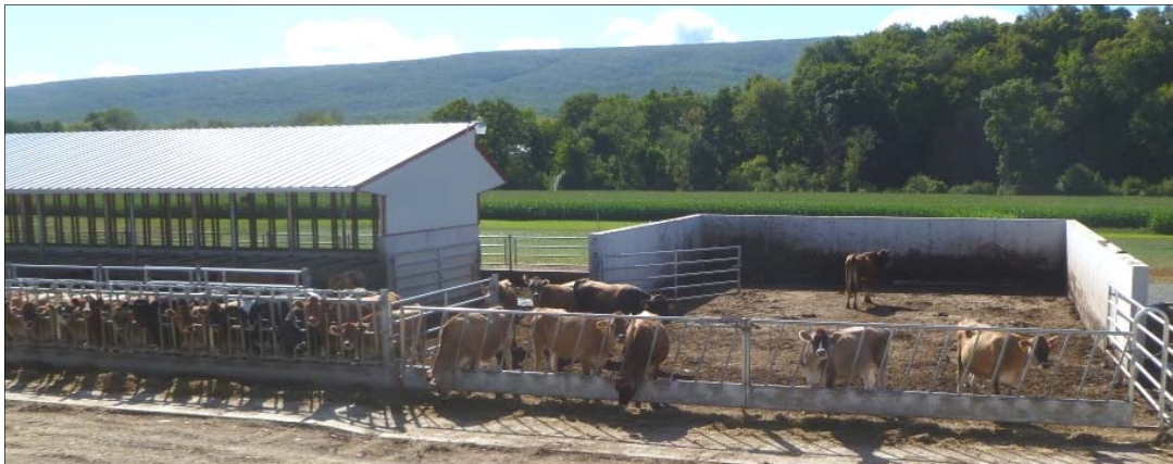
An unroofed manure stacking area with concrete walls serving a concrete cattle barnyard and lot. (left)
