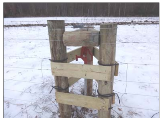
A frost free hydrant located in a pasture (right). At left, a quick disconnect for a water line where water trough portability is preferred.
