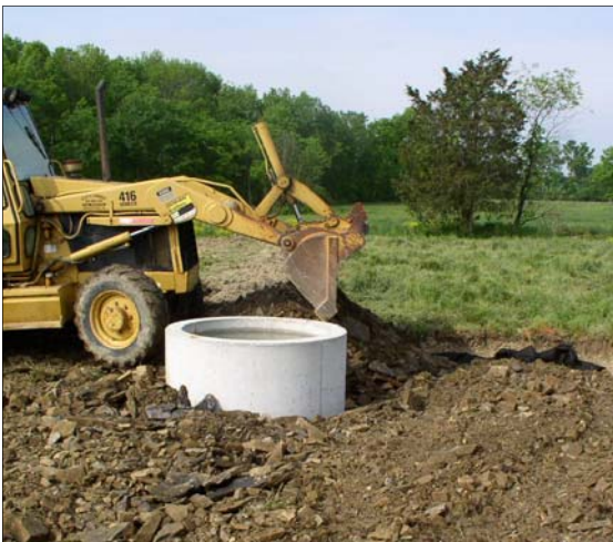
Base layer of stone being placed overtop of geotextile fabric around a precast concrete spring development trough on a dairy farm (left).
