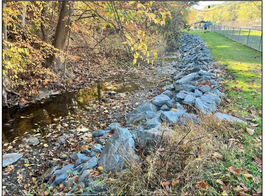
Banks along UNT to Haymaker Run stabilized with rip-rap and bank grading at Bear Hollow Park
