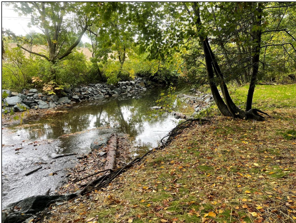
Duff Park AFTER: installation of 4 single log vane deflectors. Note the leaves and current at the end of the log structure, showing that stream flows are being directed into the middle of the channel and away from the banks.
