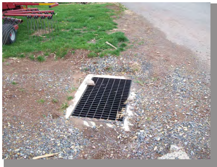
This surface inlet carries runoff and prevents scour along the existing driveway to the right.
