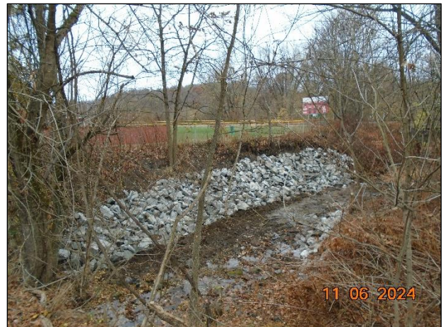
Post-construction, stabilized streambank with riprap
