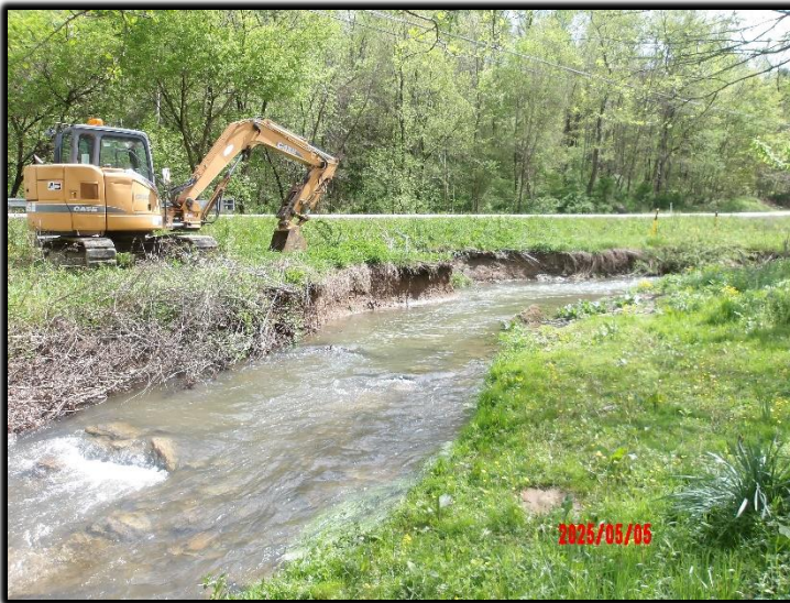
Before: Streambank erosion threatening utilities.
