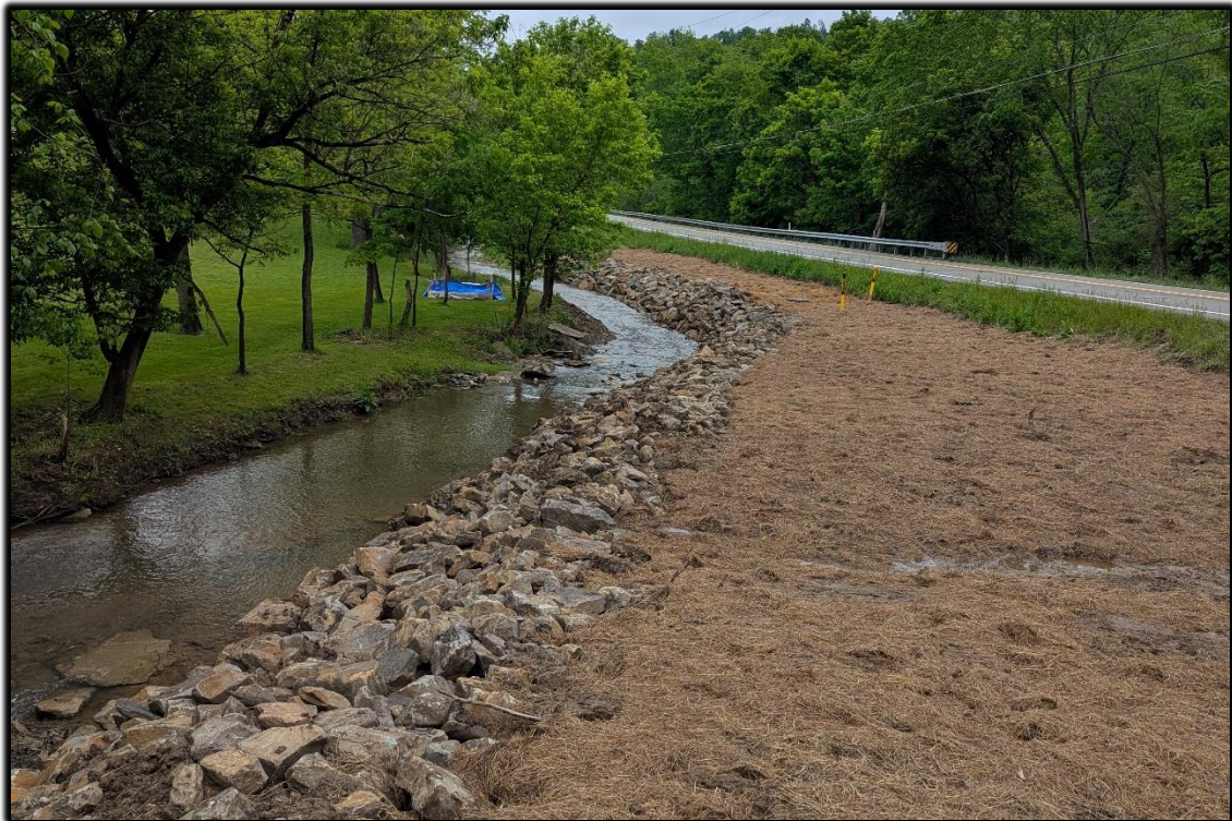
After: Stabilized streambank and yard area restored.
