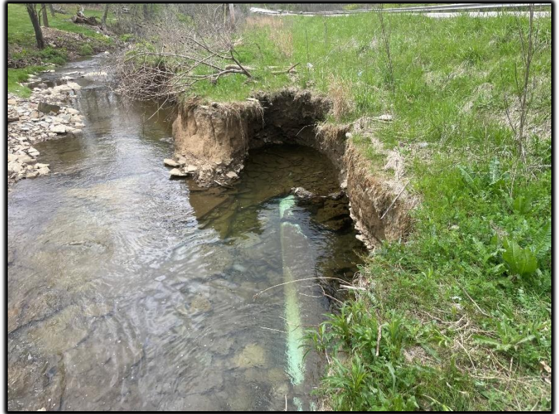
Severe streambank erosion around exposed sanitary sewer and threatening SR 366/ Greensburg Road.
