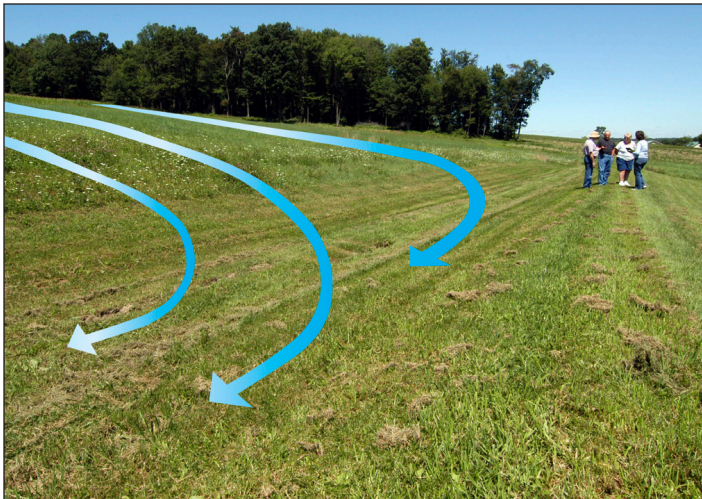
This diversion helps direct stormwater runoff from a large field away from buildings and pastures.
