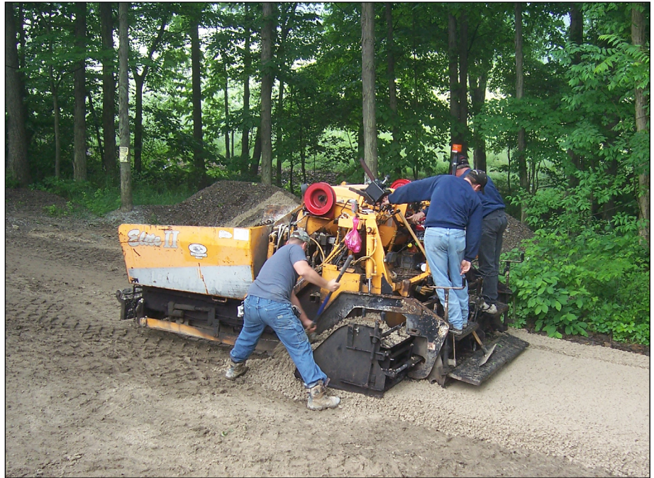
DSA being applied to Bailey's Road.
