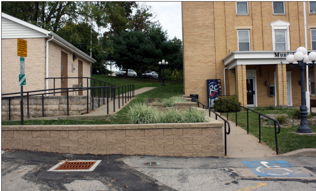
A tiered rain garden created with a concrete unit wall system keeps water from running onto the nearby pavement.
