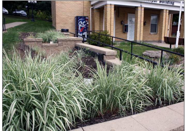
A decorative grass fills the rain garden, but the stepped weir between the upper and lower rain garden cell can be seen.
