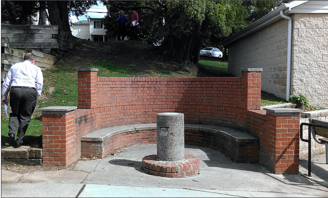
An old and broken water fountain niche in the park next to the Borough building where rain water runs off a hillside, is an opportunity for stormwater management.
