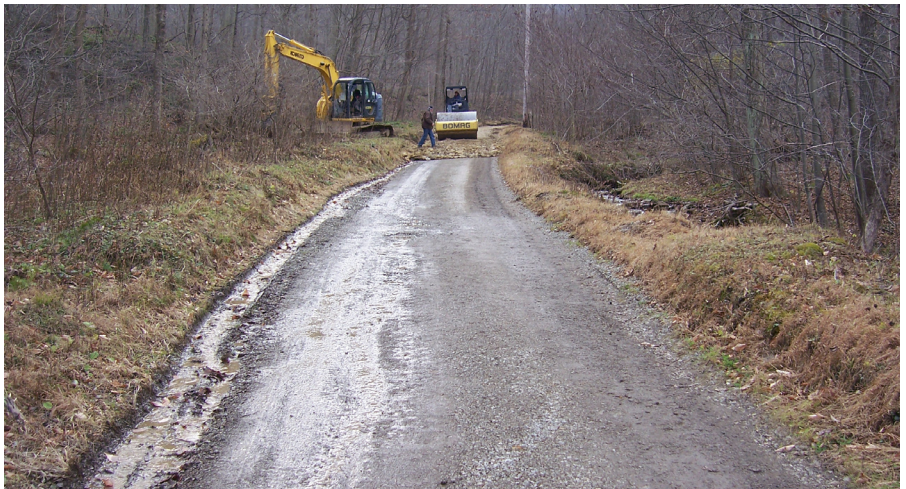
Keiper Road during construction
