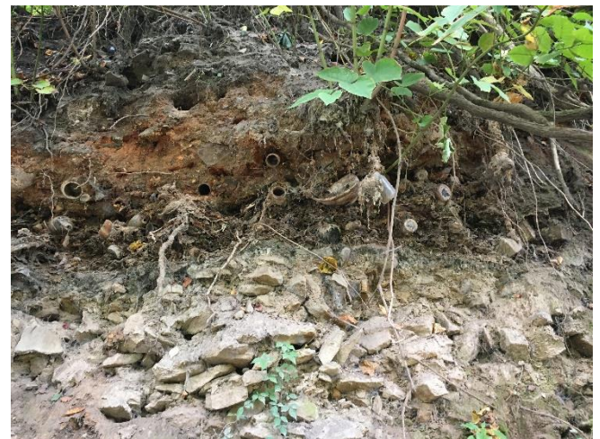
BEFORE CONSTRUCTION: Note old glass bottles sticking out of the stream banks.
