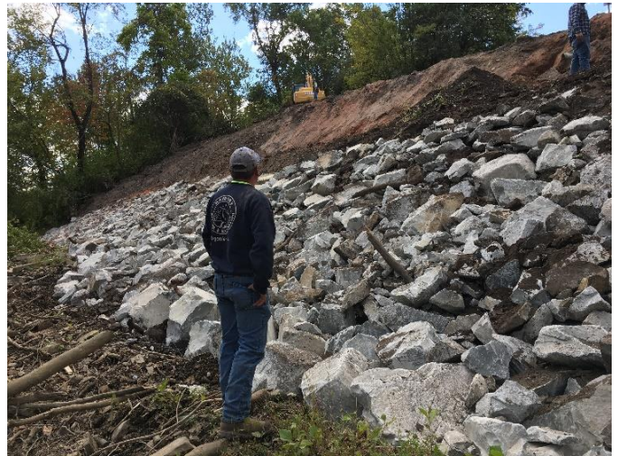
DURING CONSTRUCTION: Toe of slope armored with rip-rap.
