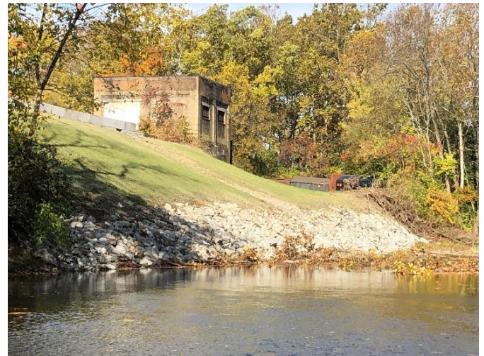
AFTER CONSTRUCTION: Stable slope.
