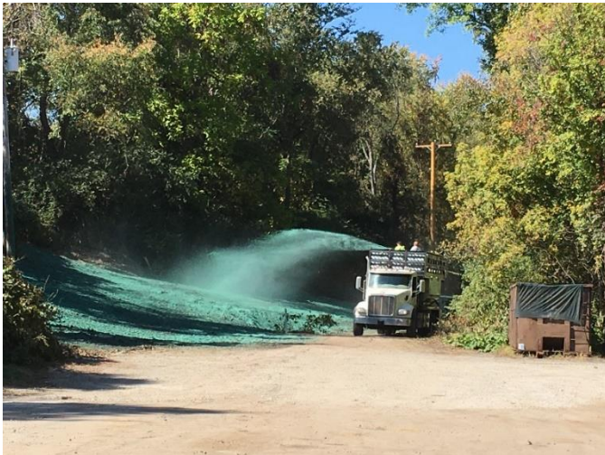
DURING CONSTRUCTION: Hydro-seeding the slope.
