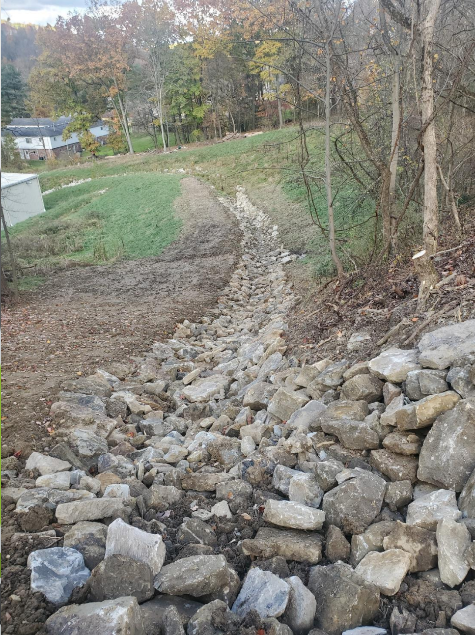
New rock-lined channel
