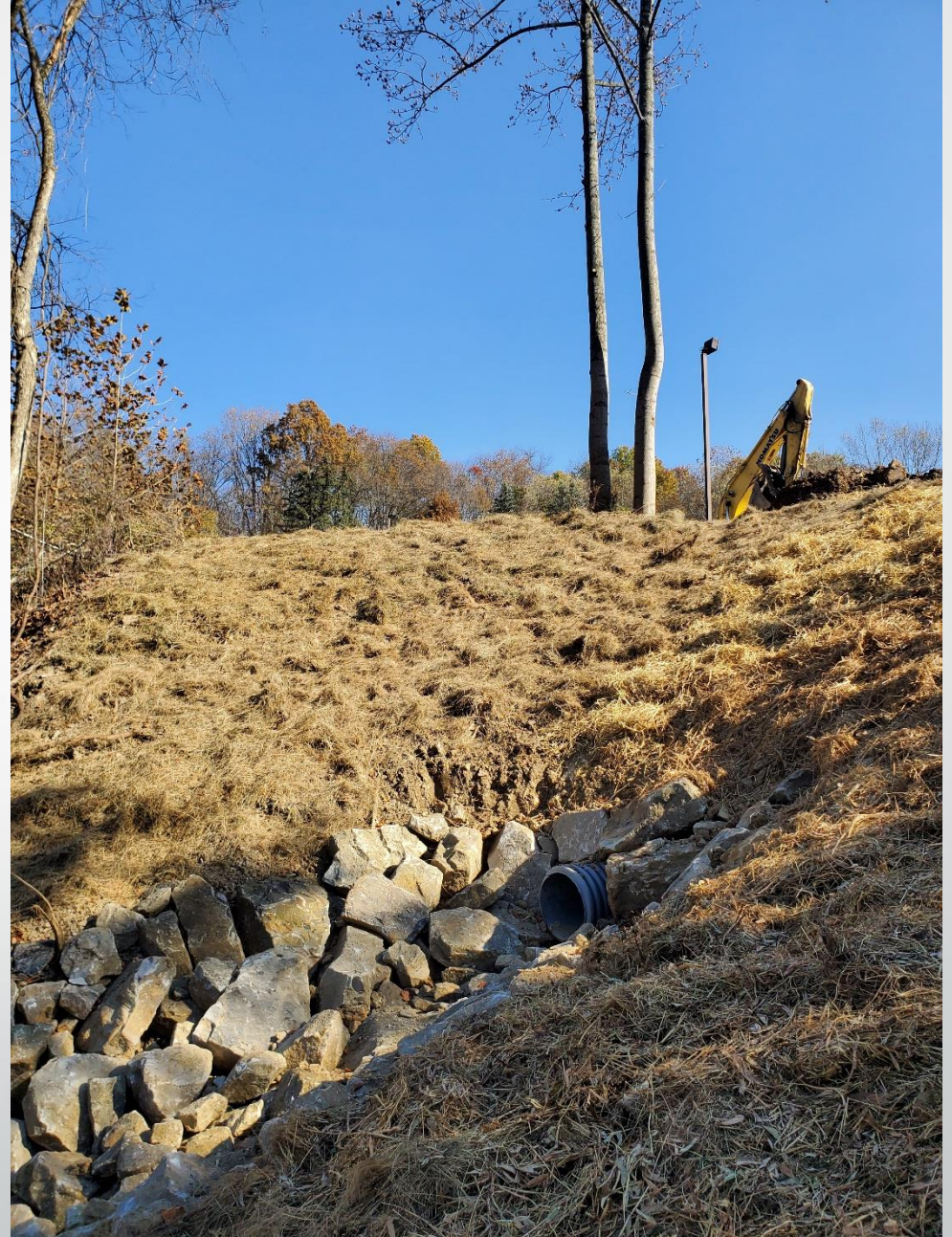
Pipe replacement and beginning of channel
