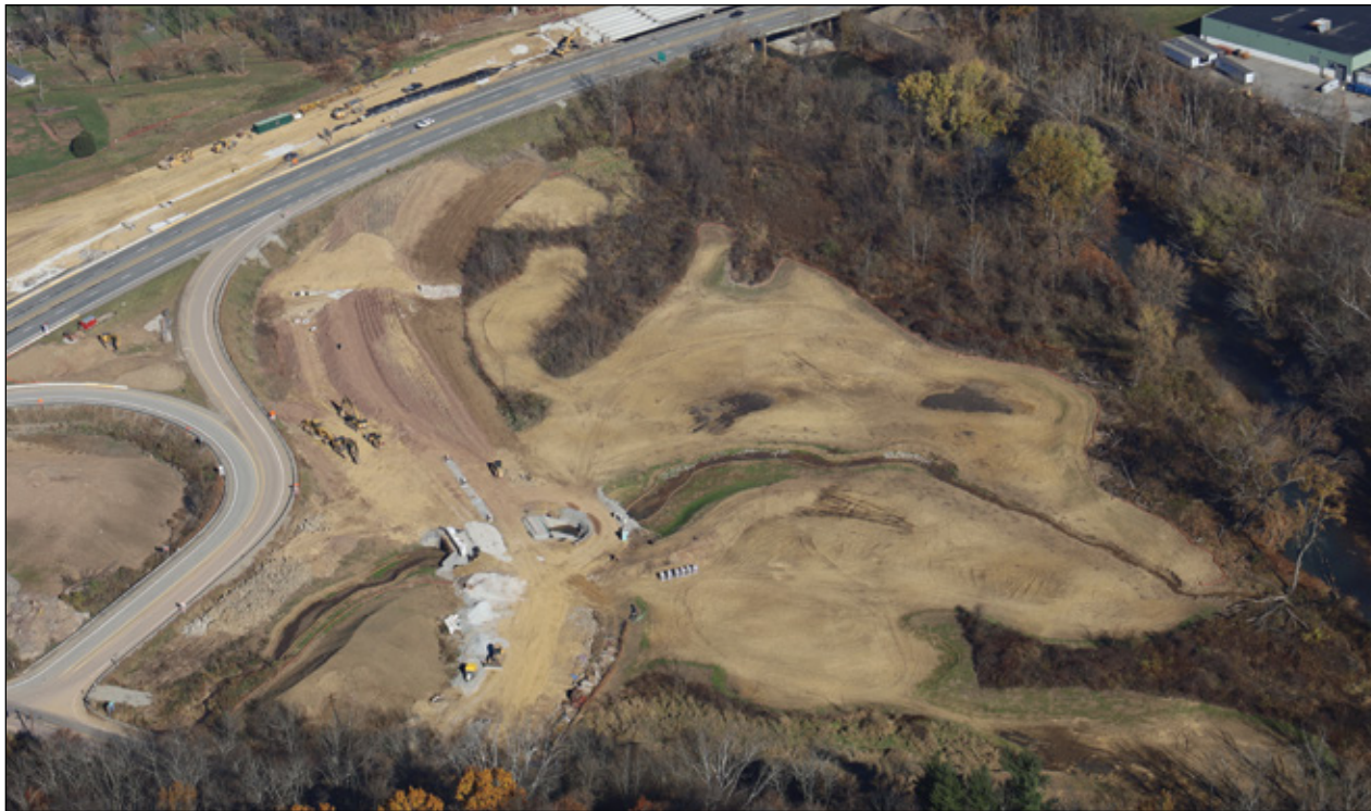
A six-acre wetland was created near Huntingdon Road to mitigate the impact of moving a portion of a stream to create a new ramp on Interstate 70. Additional mitigation efforts from this highway project will be undertaken to improve the stream in Cedar Creek Park (see pages 17-18).
