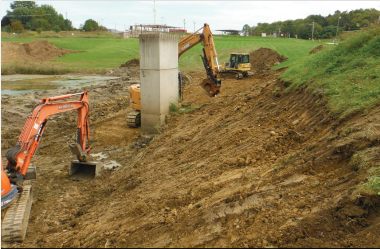
A number of existing basins in Hempfield Township were retrofitted during the year to improve their ability to manage stormwater. Left – Capacity is increased and the outlet structure is stabilized with some minor excavation. Right – Reducing the size of the outlet will allow the full capacity of the basin to be used during large storms.
