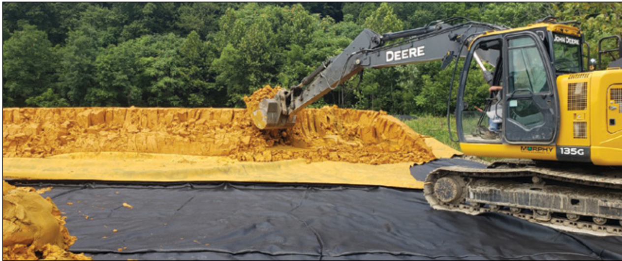
At the Lowber mine-discharge treatment site, an excavator is used to stir the iron sludge to speed its drying. Iron oxide is a pollutant that drops out of the mine water as it flows through the site's holding ponds. Periodically, it is removed from the ponds and stored on-site until it is dry enough to truck away.
