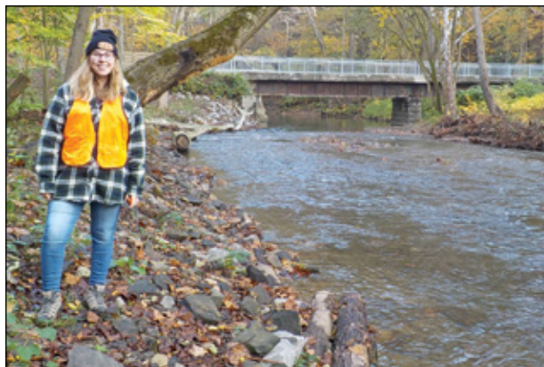
A large mudsill was installed to stabilize this area of streambank along Turtle Creek, and reduce the undercutting of a bridge abutment that carries the Westmoreland Heritage Trail over the stream (background).
