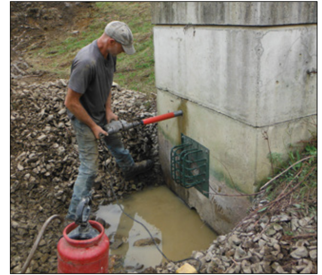
A number of existing basins in Hempfield Township were retrofitted during the year to improve their ability to manage stormwater. Left – Capacity is increased and the outlet structure is stabilized with some minor excavation. Right – Reducing the size of the outlet will allow the full capacity of the basin to be used during large storms.
