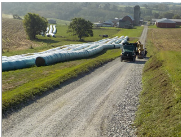
Before (left) and after (right) improvements to a one-half-mile stretch of Helen Road in Salem Township. The profile of this low-volume road, near Crabtree Creek, was raised by adding some 1,000 tons of fill. More than 1,000 feet of underdrains also were installed.
