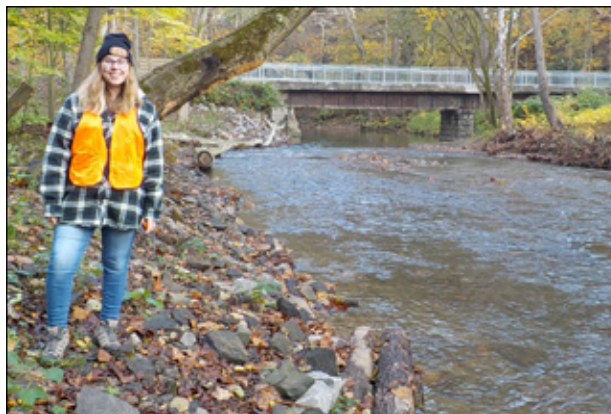
A large mudsill was installed to stabilize this area of streambank along Turtle Creek, and reduce the undercutting of a bridge abutment that carries the Westmoreland Heritage Trail over the stream (background).
