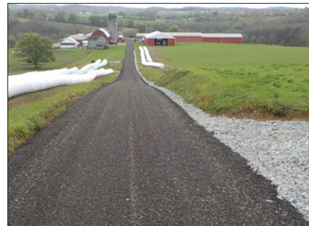
Before (left) and after (right) improvements to a one-half-mile stretch of Helen Road in Salem Township. The profile of this low-volume road, near Crabtree Creek, was raised by adding some 1,000 tons of fill. More than 1,000 feet of underdrains also were installed.
