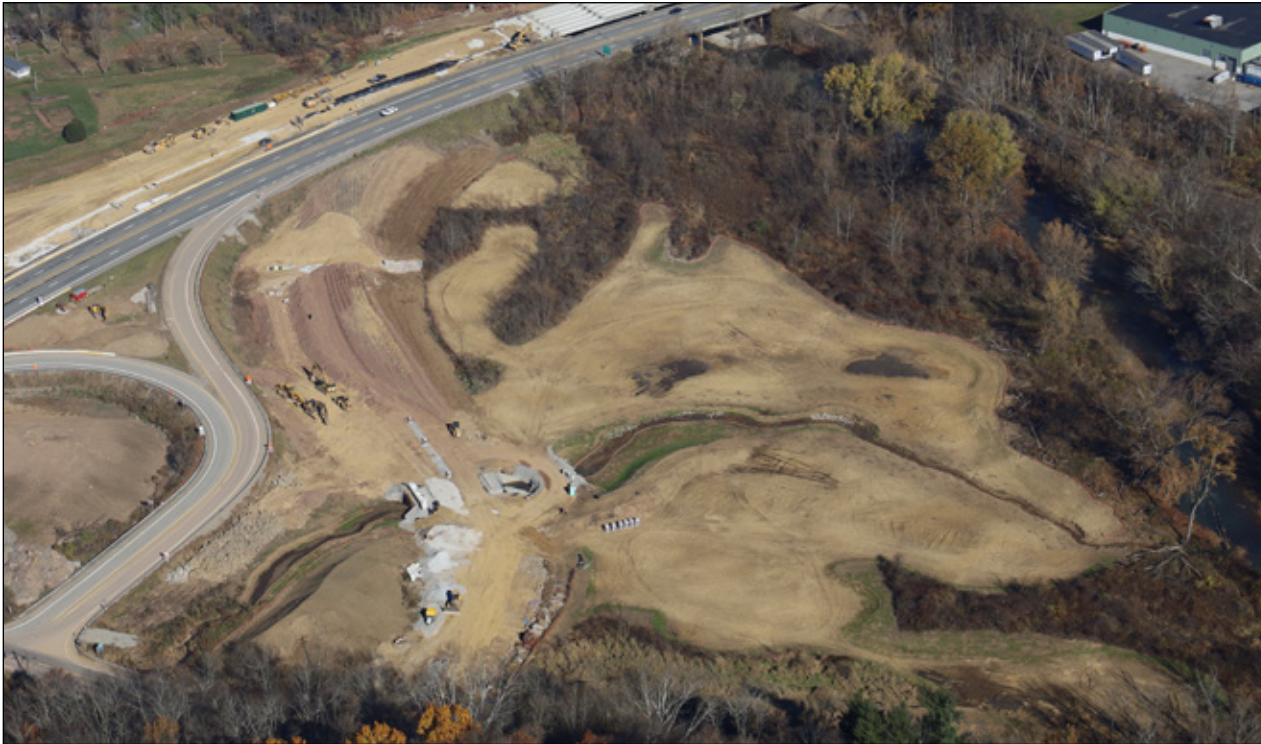
A six-acre wetland was created near Huntingdon Road to mitigate the impact of moving a portion of a stream to create a new ramp on Interstate 70. Additional mitigation efforts from this highway project will be undertaken to improve the stream in Cedar Creek Park (see pages 17-18).
