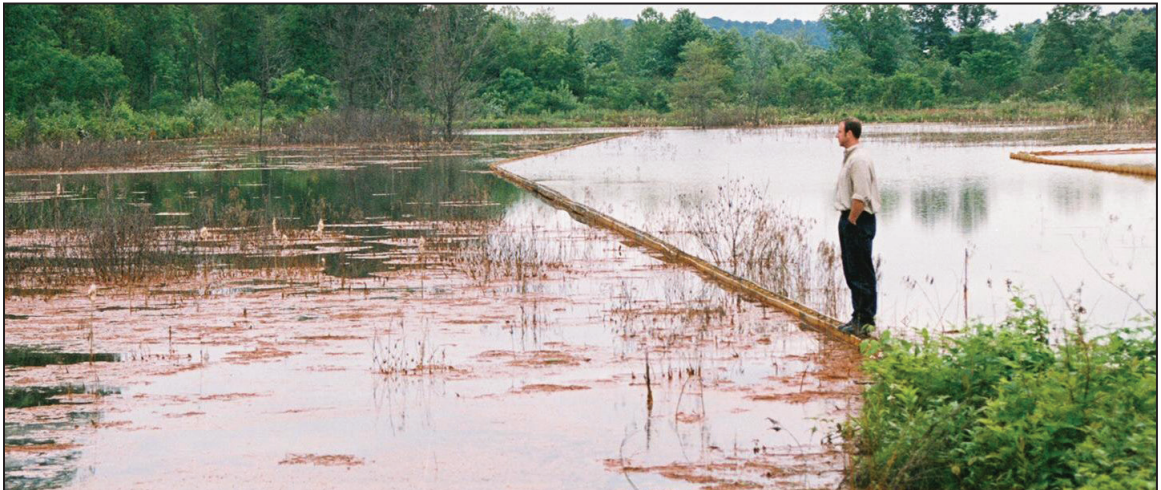
Westmoreland Conservation District/CEO Manager Rob Cronauer visits the Brinkerton Abandoned Mine Drainage Treatment System in the Sewickley Creek Watershed.
