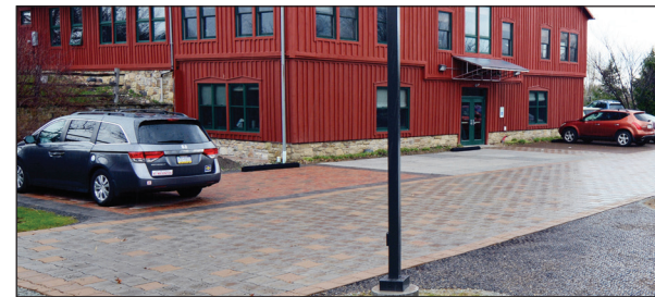
Several different kinds of permeable pavers were used in the barn's back parking lot for demonstration purposes.
