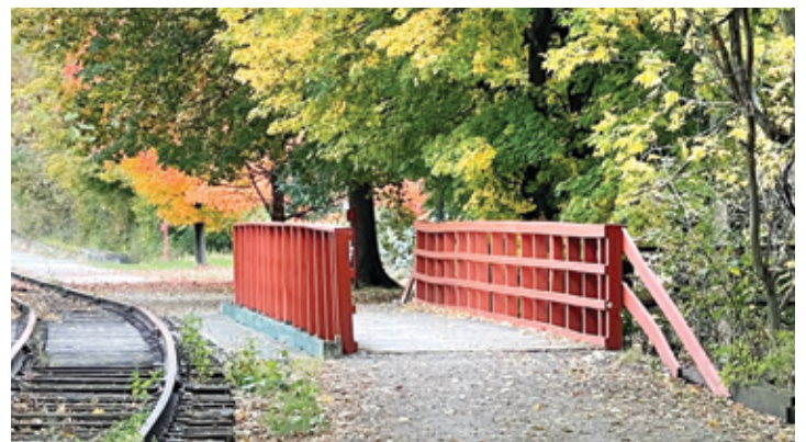
The Pittsburgh Street Bridge in The City of Greensburg
