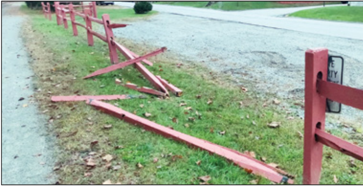
Vandalized fence at the Willow Crossing Access Area
