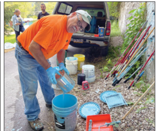
Longtime volunteer Malcolm Sias gathers tools and what's left of the light blue paint.
