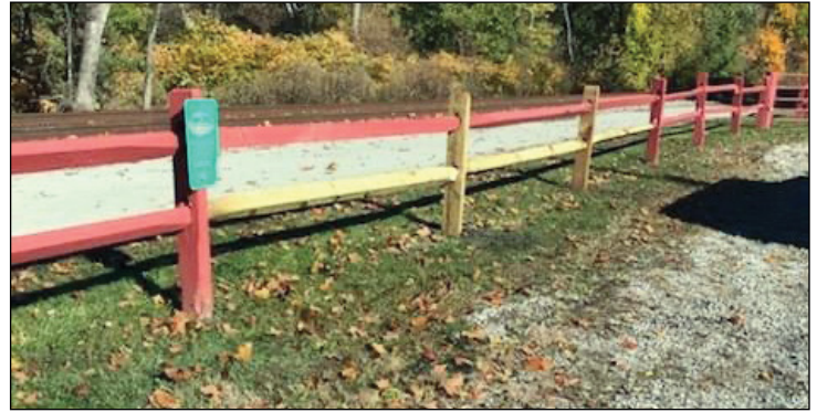
Repaired and restored by our trail maintenance volunteers.
