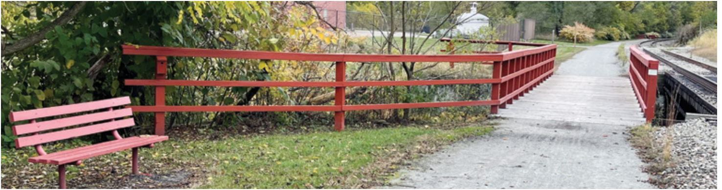
Logan Williams and his team stained the fence, rails and bench at the bridge over Jack's Run in South Greensburg.
