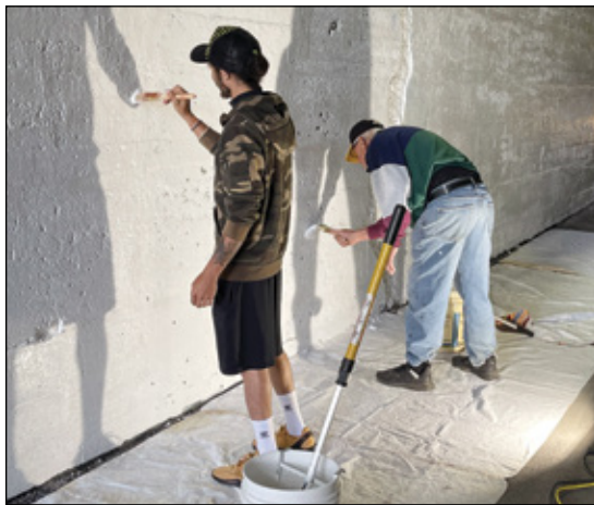
Applying the white primer over the old mural with drop cloths in place.
